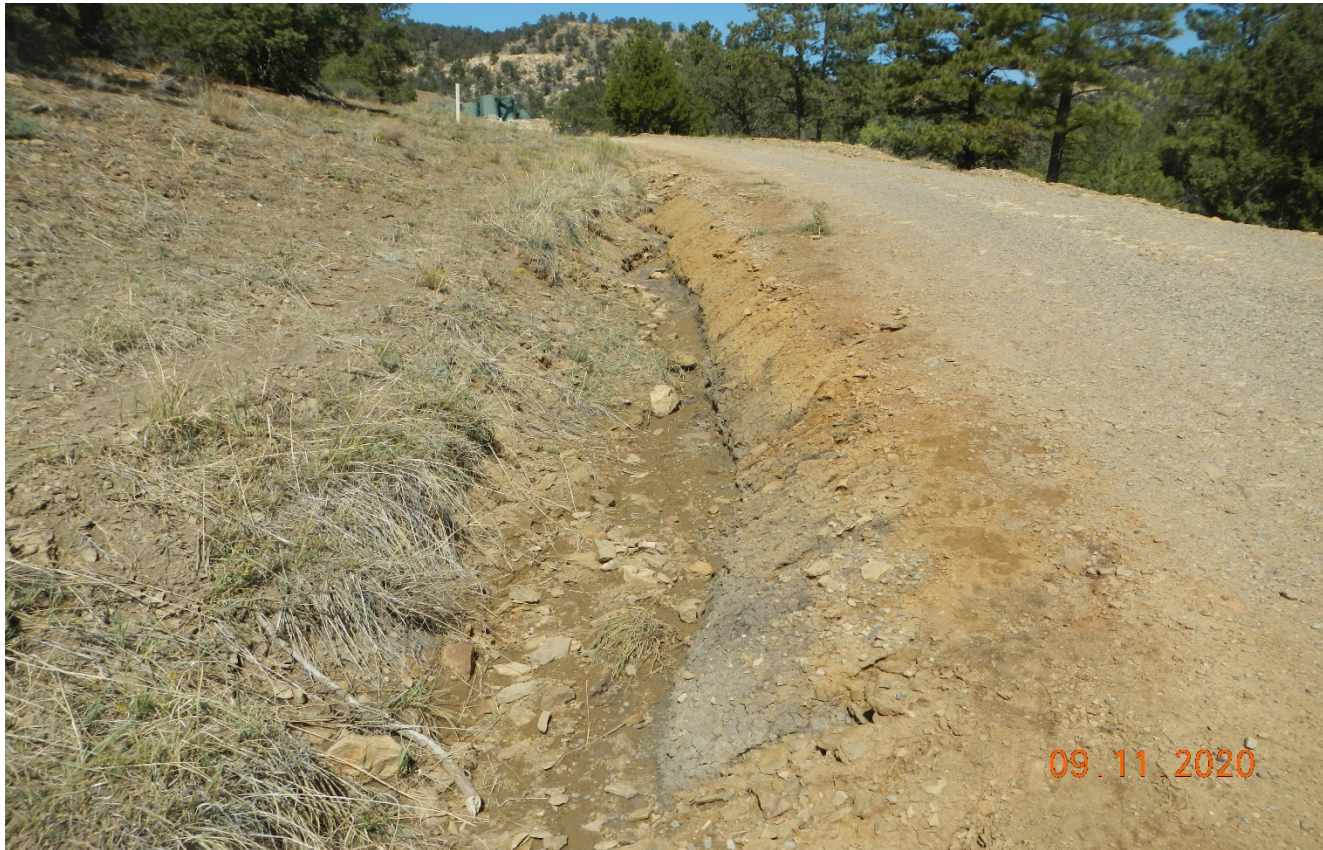
Photo 4. There is erosion along the side of the road that needs to be repaired and stabilized.
