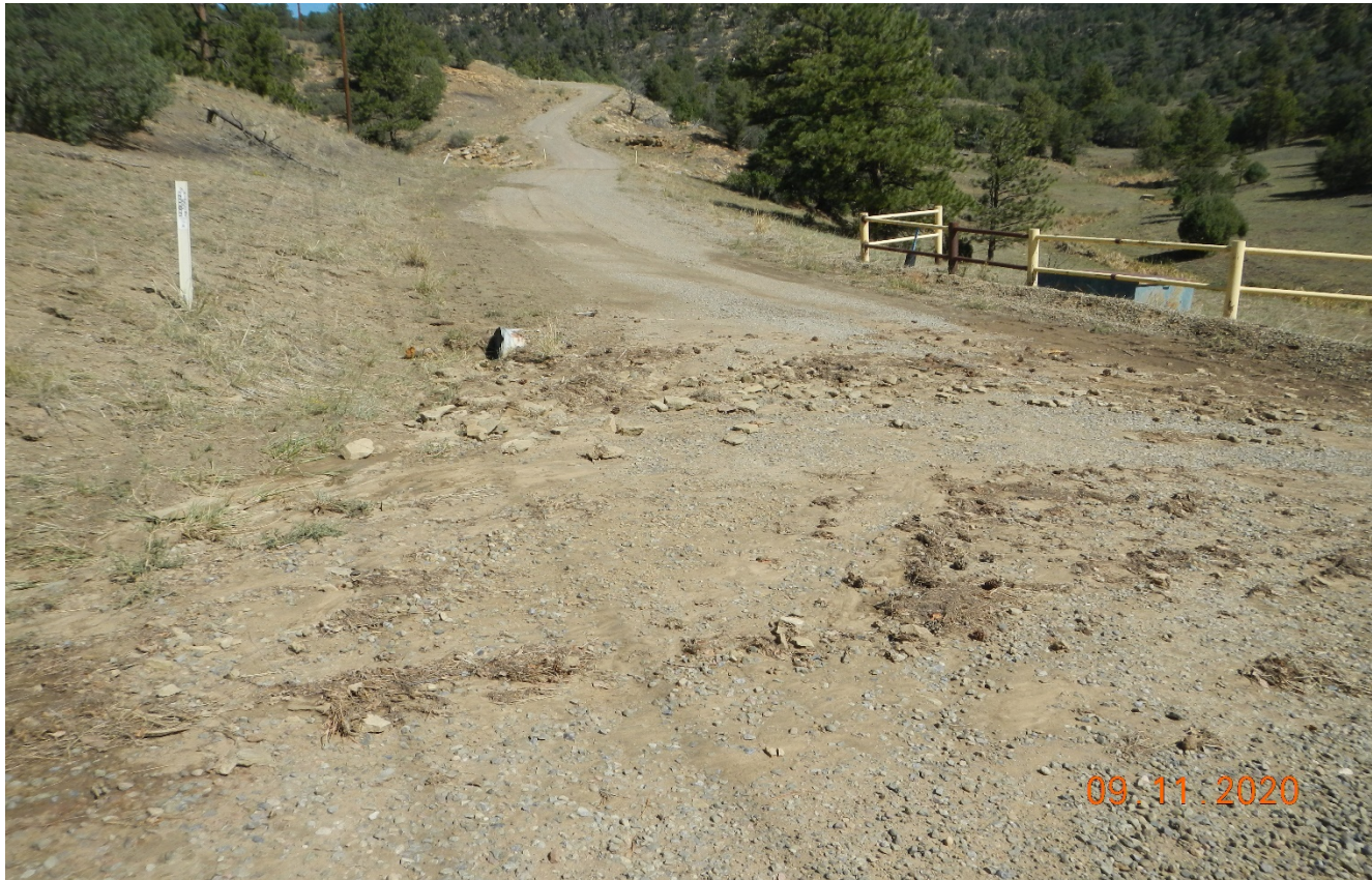
Photo 2. Stormwater is not properly diverted toward the culvert.
