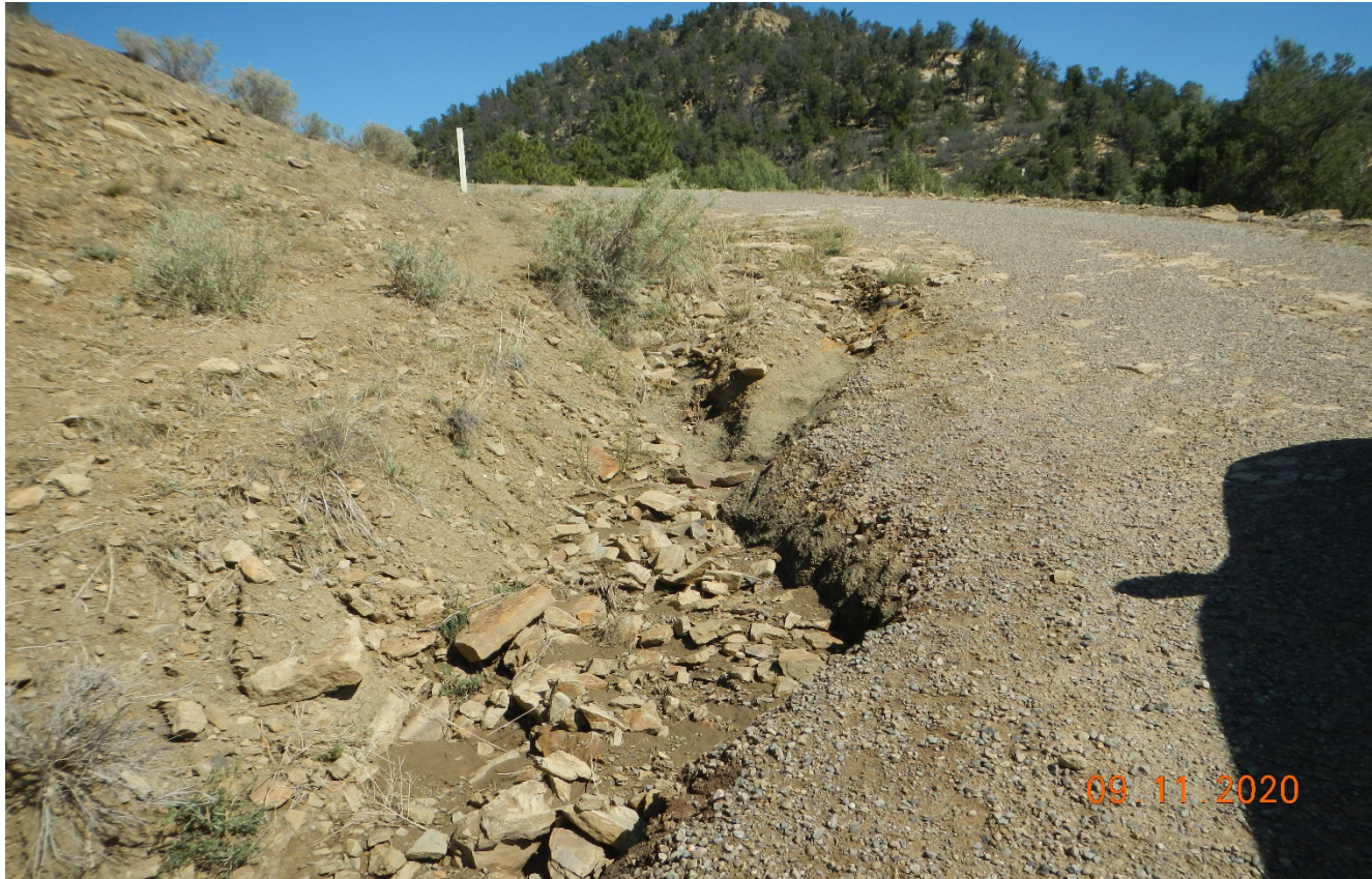
Photo 3. There is erosion along the side of the road that needs to be repaired and stabilized.
