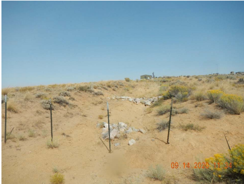
Photo 7. Erosion from location down to access road. Photo on access road looking towards location.
