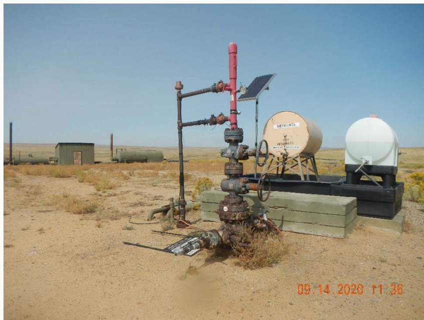
Photo 3. Wellhead sign knocked over. Hissing at wellhead.
