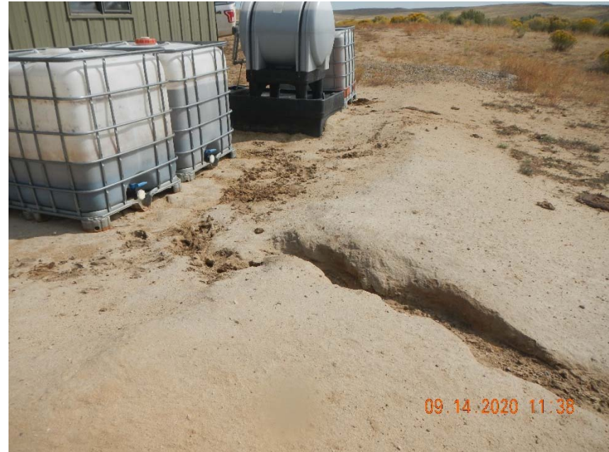
Photo 8. Erosion from location down to access road. Photo taken on location.
