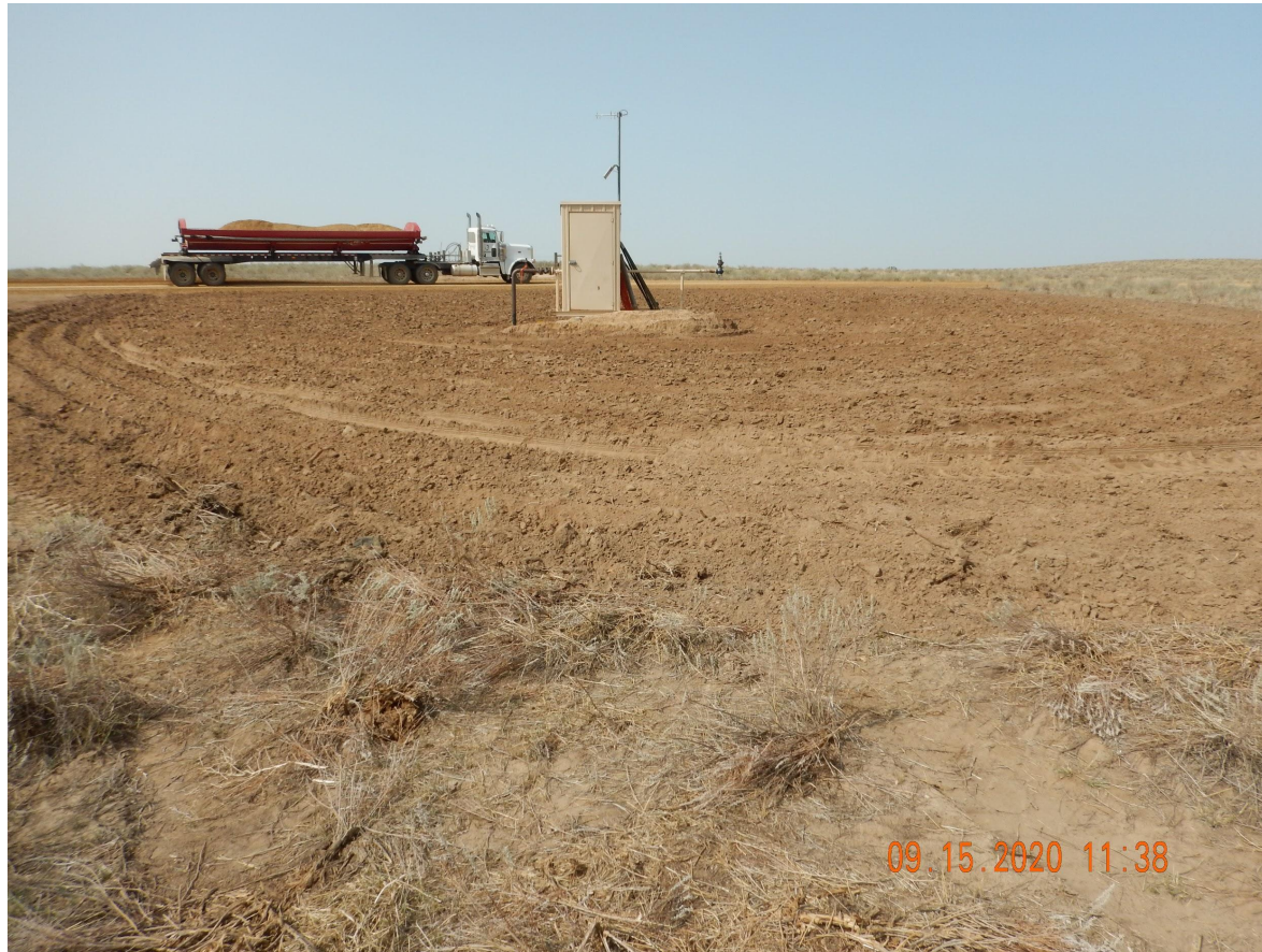
Photo 2. Photo taken from the associated offsite tank battery location, facing West. Photo illustrates the Operator has decommissioned the tank battery. Equipment, meter house, still remains at the location. In addition, final reclamation activities have been initiated by removing gravel and performing compaction alleviation.
