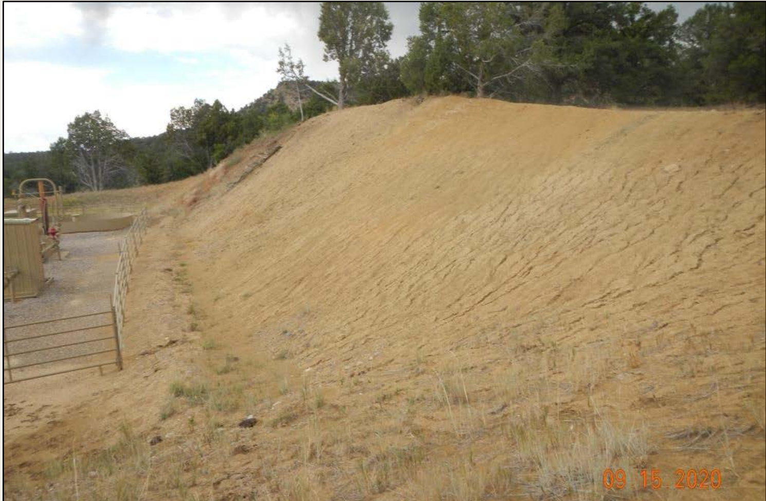
Photo 3. View of bare soils on the northern cut-slope. Erosion controls are needed here.
