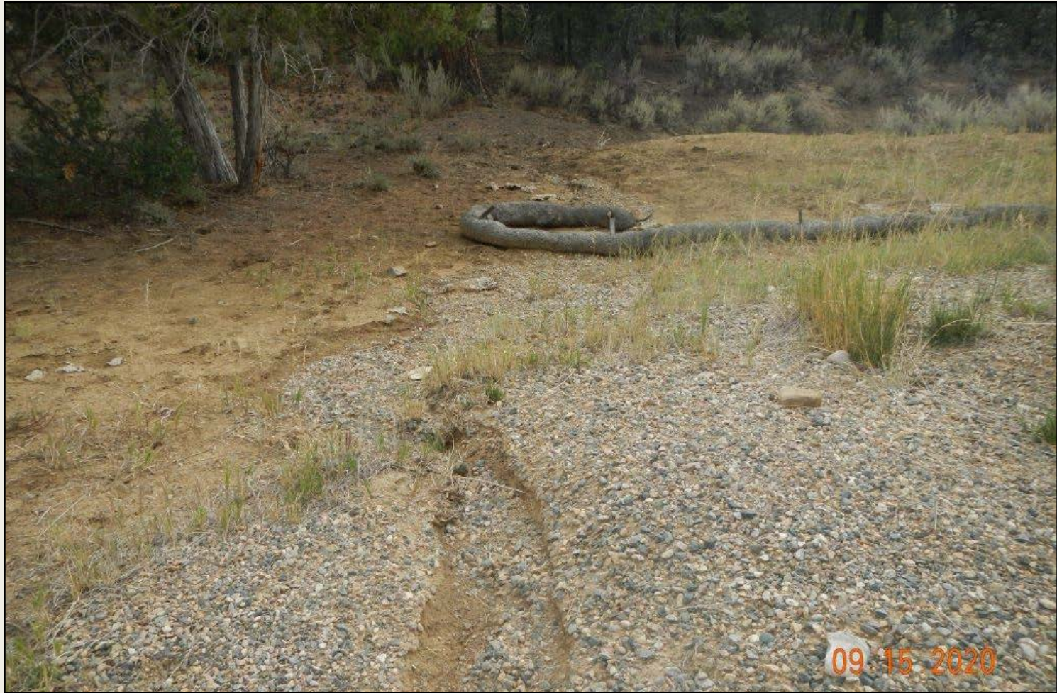
Photo 2. View of erosional channel (approx. 1 ft wide and 6-8 in deep) in the southeastern project area and wattle needing repair /maintenance.
