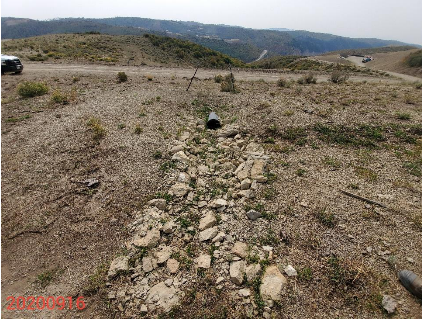
Photo 5: Photo shows sediment trap and culvert on the north end of the Location
