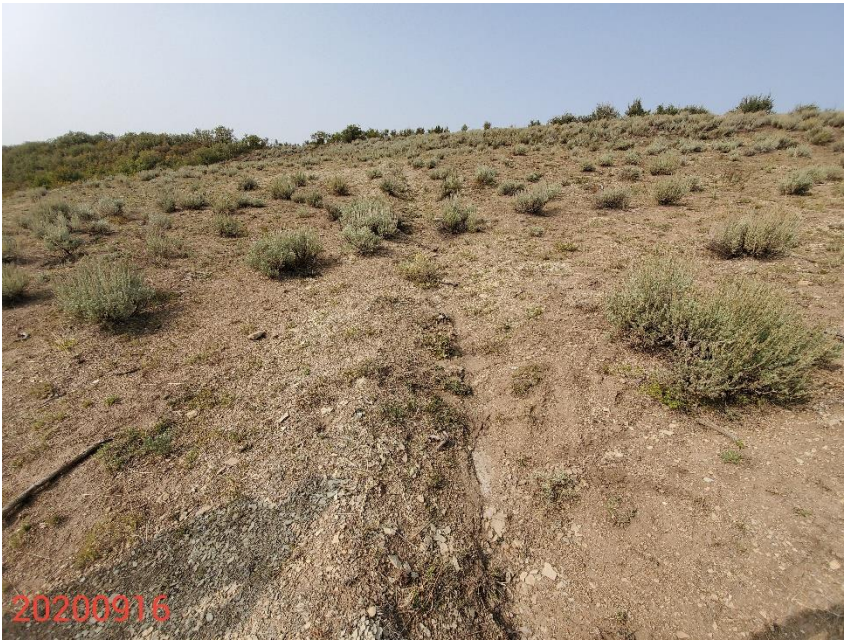
Photo 3: Photo taken from one of the stormwater ditches on the Location, facing southwest. Stormwater channelization and cutting within the ditch is becoming evident and Operator is advised to implement BMPs in conjunction with the ditches to alleviate stormwater velocity within the ditch, to mitigate further incising within the ditch.
