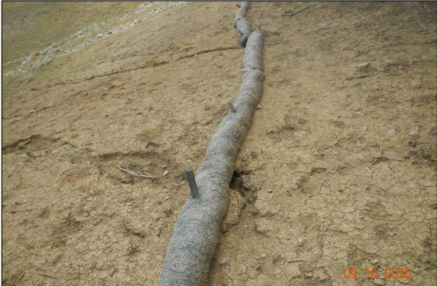
Photo 3. View of BMPs on the northwestern edge of the project area, needing maintenance.
