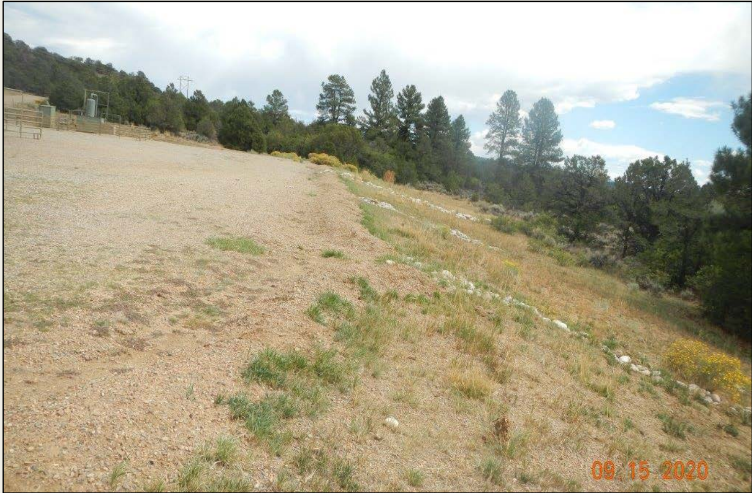
Photo 2. View of the southern fill slope from the southwestern corner facing eastward. Revegetation is progressing within the interim reclamation area, largely with grasses such as western wheatgrass and sand dropseed.
