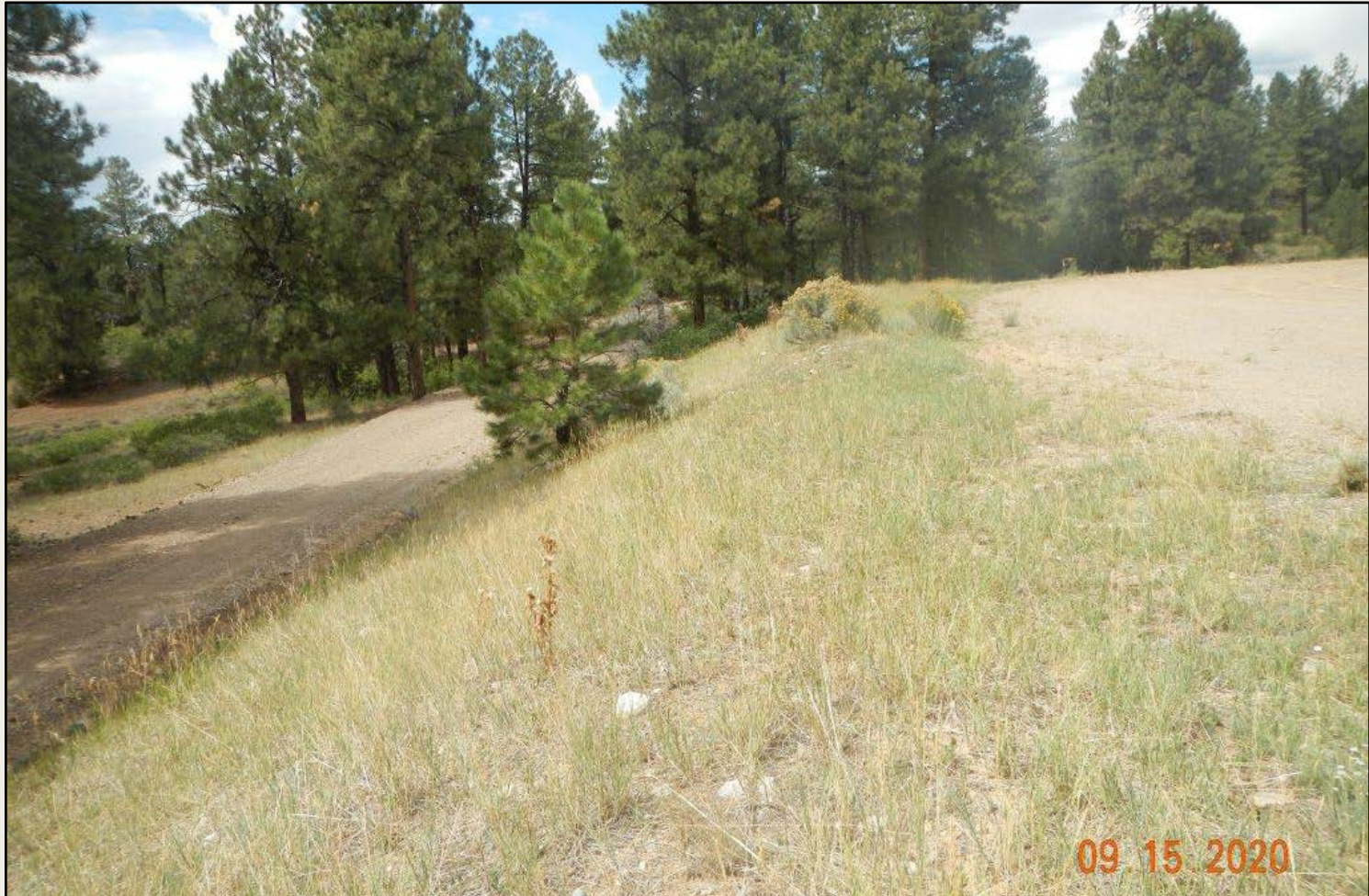
Photo 2. View of the western fill slope from the southeastern corner facing northward. Revegetation is progressing within the interim reclamation area, largely with grasses such as western wheatgrass and sand dropseed.
