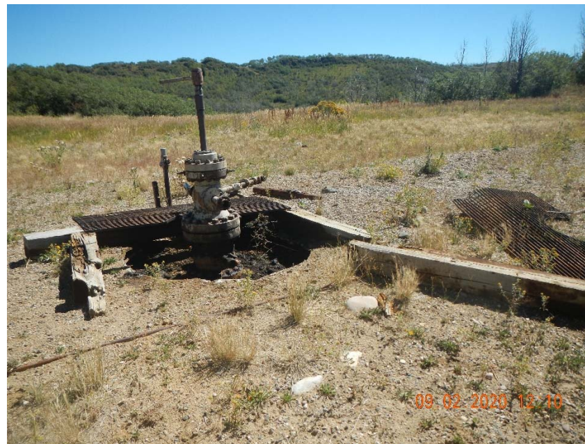
Photo 2. Stained soil at wellhead.
