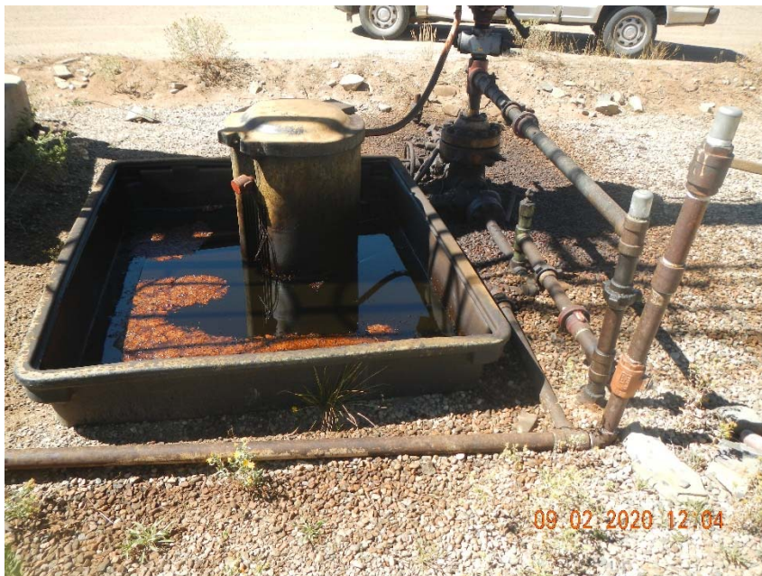
Photo 3. Stained soil at wellhead, secondary containment with oily fluid.
