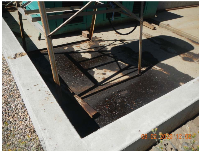
Photo 8. Stained concrete in tank battery berm.
