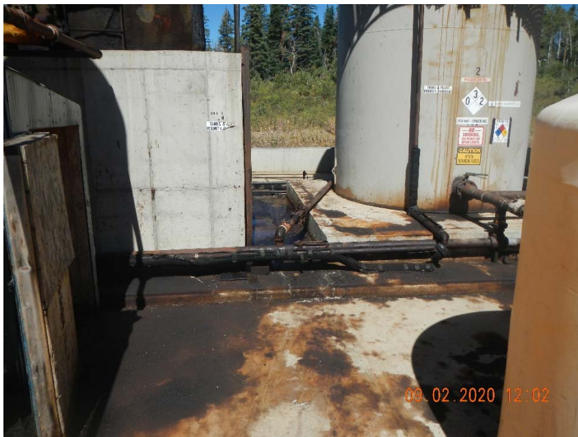
Photo 7. Stained concrete in tank battery berm.
