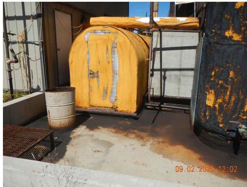
Photo 6. Stained concrete in tank battery berm.
