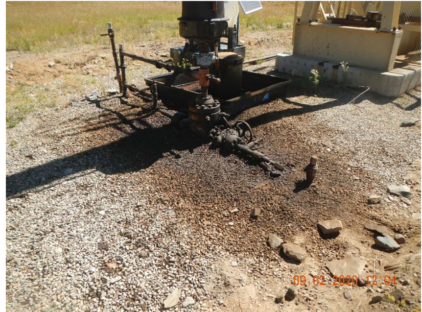
Photo 2. Stained soil at wellhead. Fresh gravel with staining coming through around perimeter.
