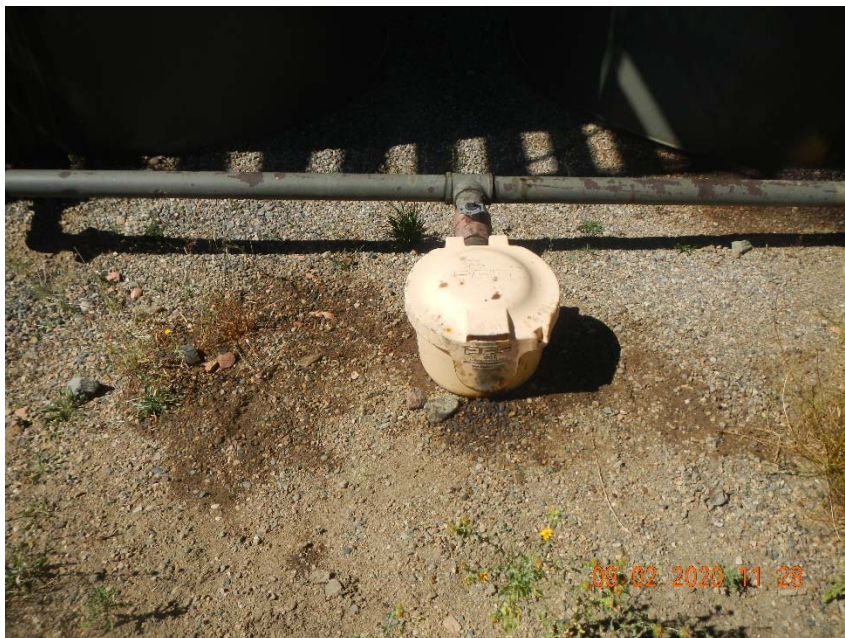
Photo 5. Close up of soil staining at loadout.
