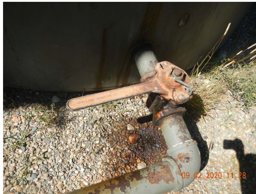
Photo 8. Close up of soil staining at loadout.
