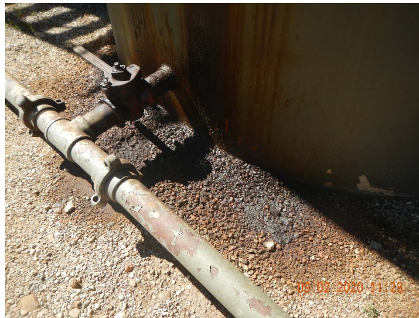
Photo 6. Close up of stained soil from tank overflow.
