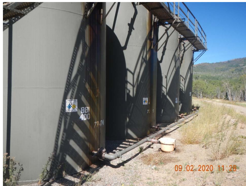
Photo 4. Stained soil from tank overflow and at loadout.
