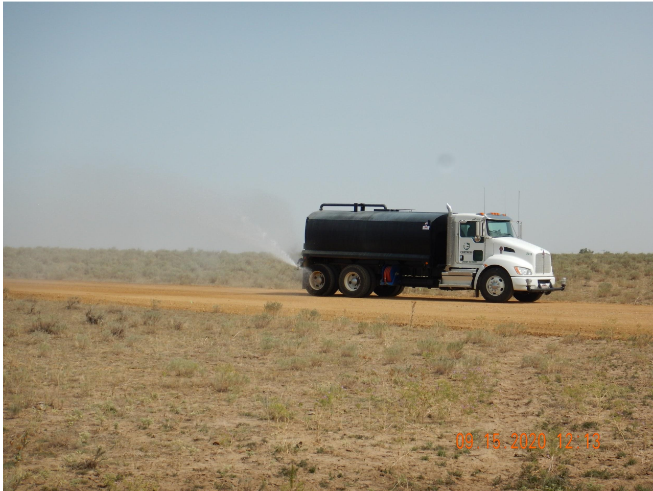
Photo 8. Photo taken from a portion of the main access road, facing North. Photo illustrates Operator had a water truck on location controlling fugitive dust.
