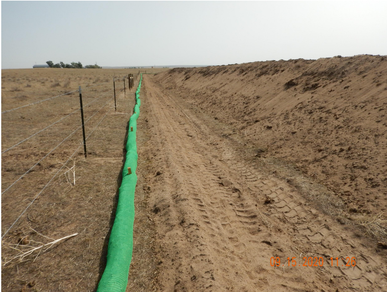
Photo 3. Photo taken from the northern location, facing East. Photo illustrates Operator has installed stormwater BMPs (ditch and berm, filtrex wattles) around the entire perimeter of location. Note: north-facing stockpile has not been stabilized. Operator indicated this would be stabilized with hydromulch and broadcast seeding.
