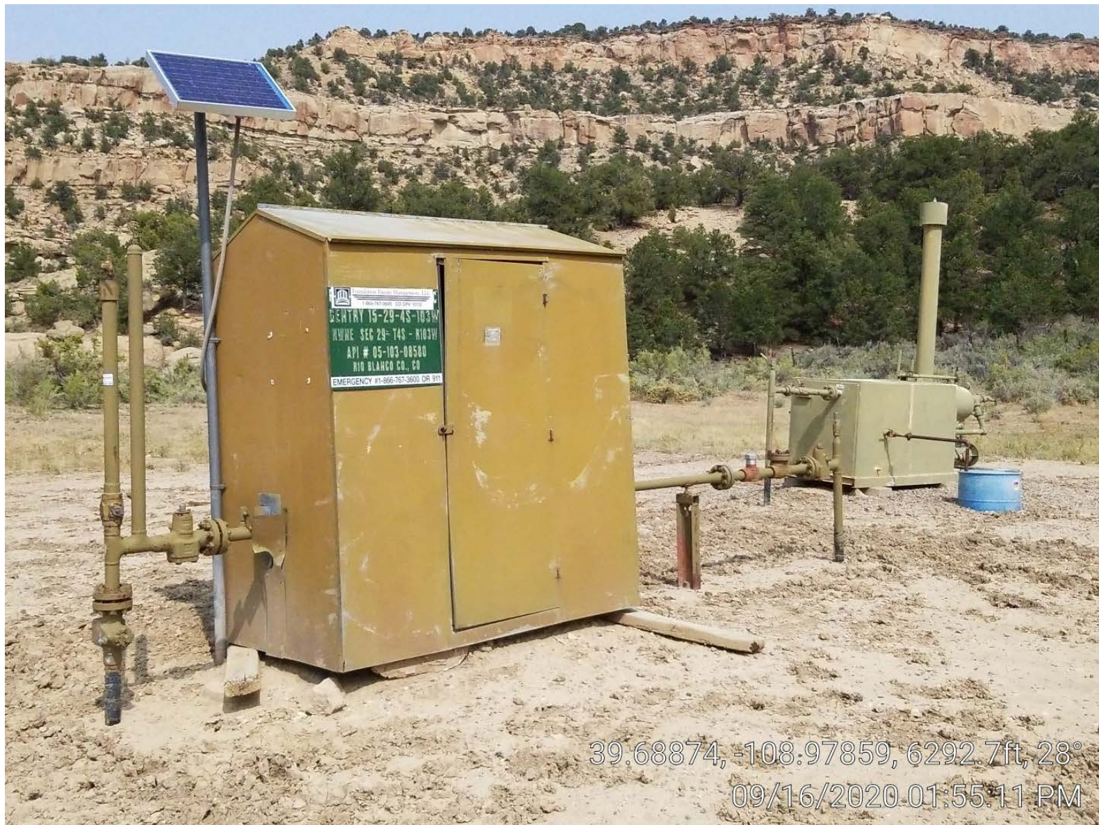
Photo 2. Meter building, tank, separator.
