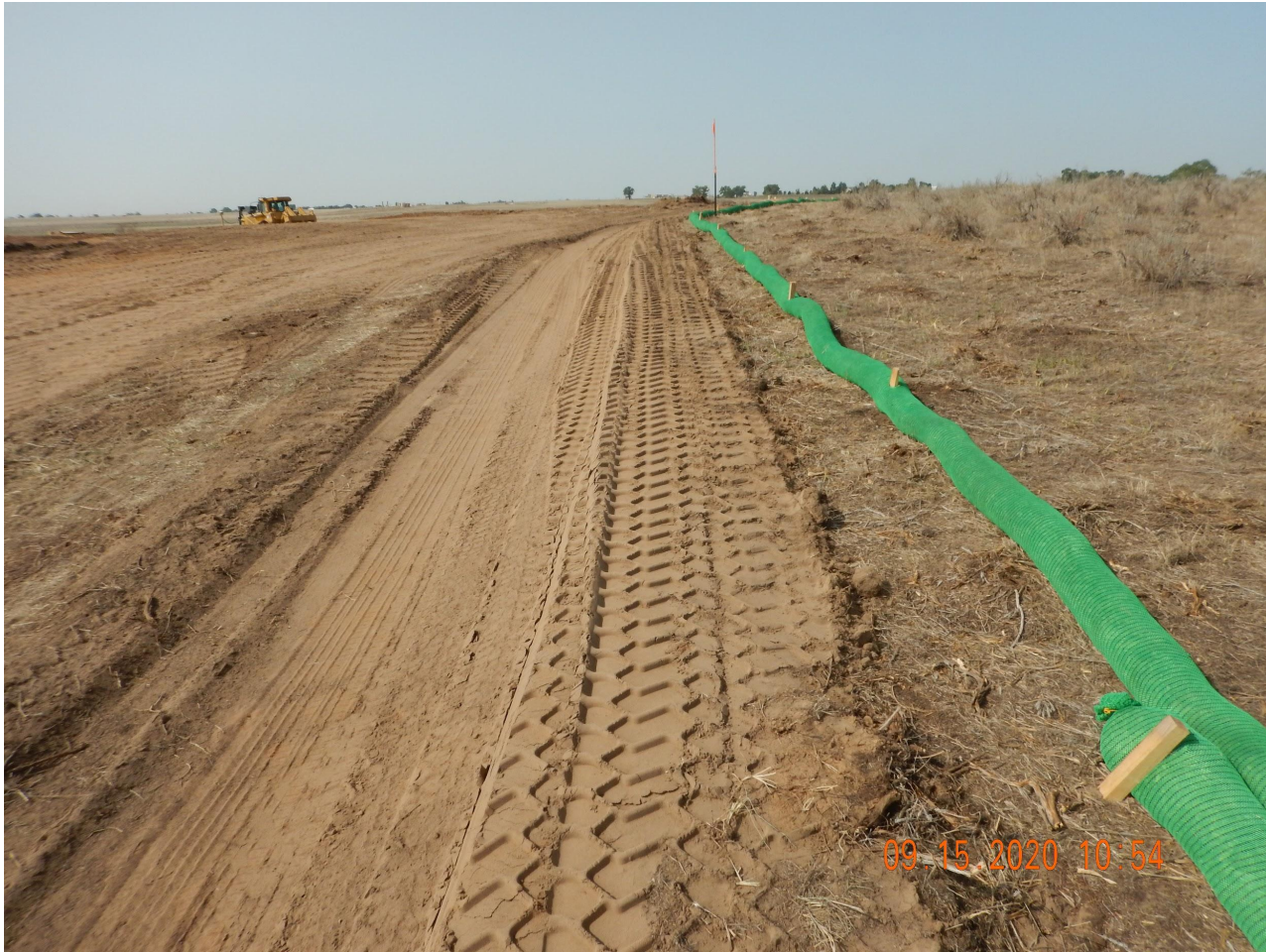
Photo 2. Photo taken from the northeastern location, facing West. Photo illustrates Operator has installed stormwater BMPs (ditch and berm, filtrex wattles) around the entire perimeter of location.
