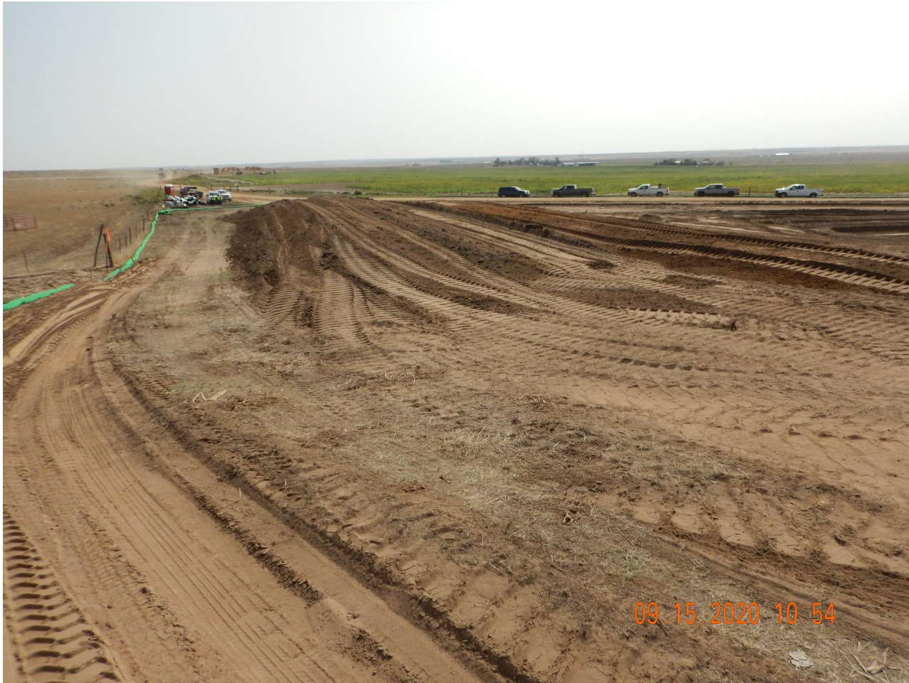
Photo 3. Photo taken from the northeastern location, facing East. Photo illustrates Operator is stockpiling topsoil along the northeastern location.
