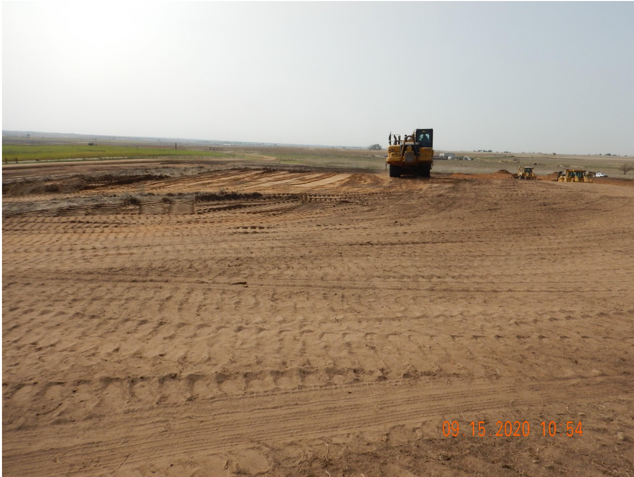
Photo 1. Photo taken from the northern location, facing South. Photo illustrates Operator is in process of performing topsoil salvage operations.
