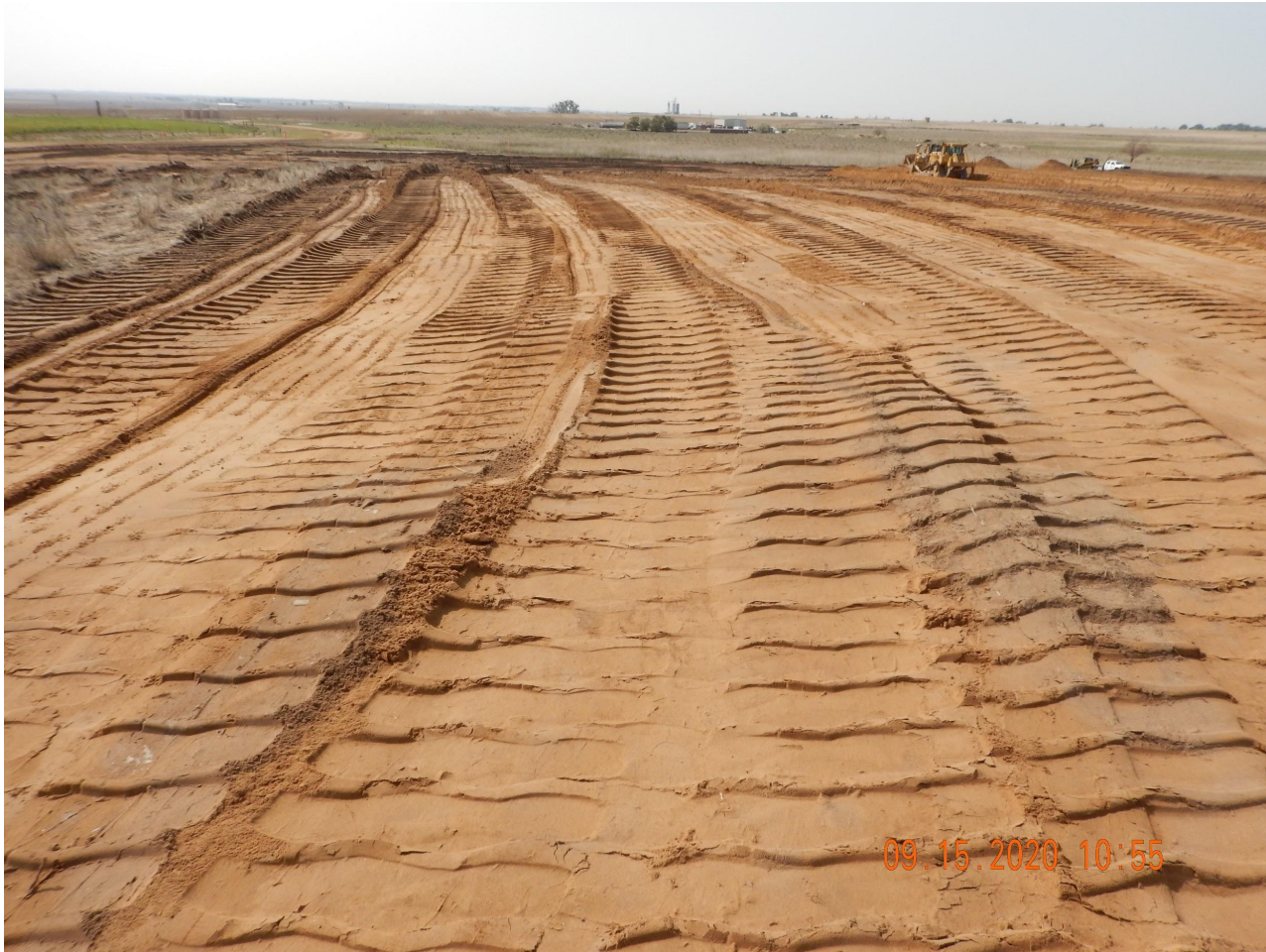
Photo 4. Photo taken from the northern section of the location, facing South. Photo illustrates Operator appears to be salvaging topsoil to an appropriate depth.
