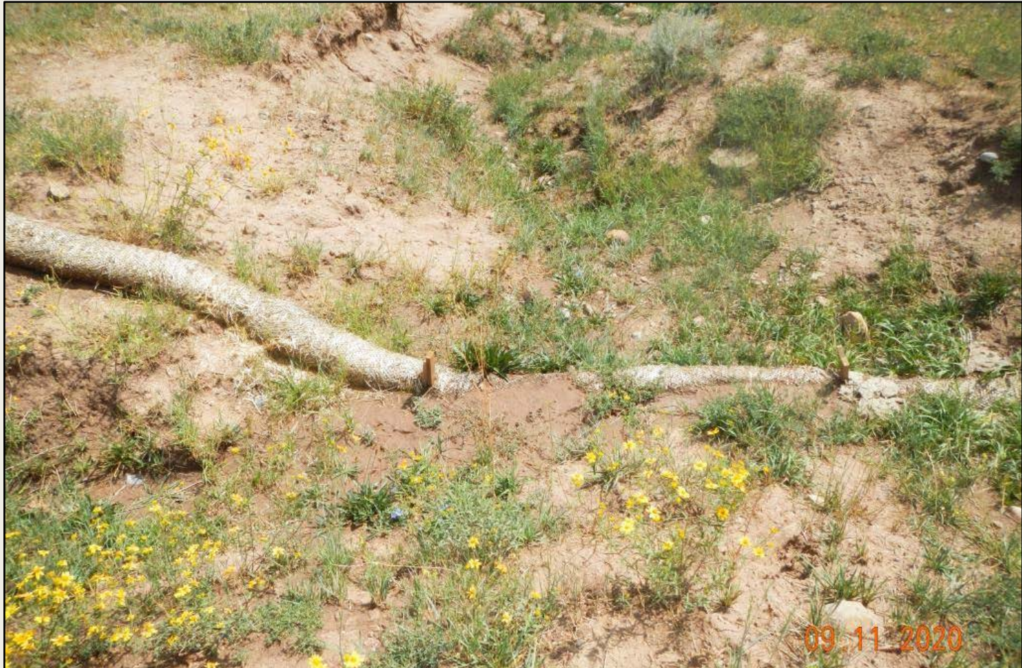
Photo 3. View of wattle in the southwestern project area that is full of sediment.
