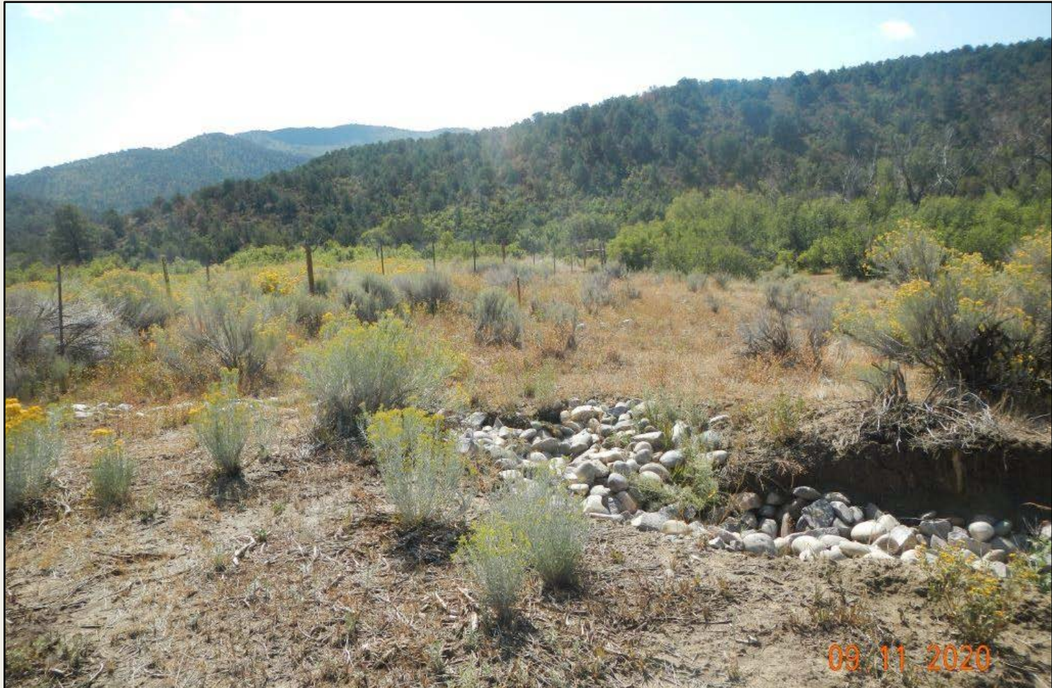
Photo 3. View of the western project area from the northwestern corner facing southward. Cobble run-down placed in erosional channel appears to be functioning. Note that smooth cobble can accelerate velocity of water flows and is not recommended as a stormwater BMP. Continue monitoring to ensure site stabilization.
