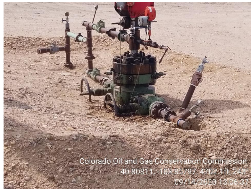
Photo 4 – 3414H Wellhead, Stained Soil
