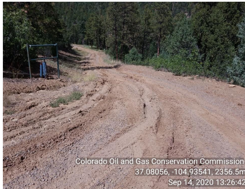
Photo 4 stormwater issues on access road from Big Bingham main road
