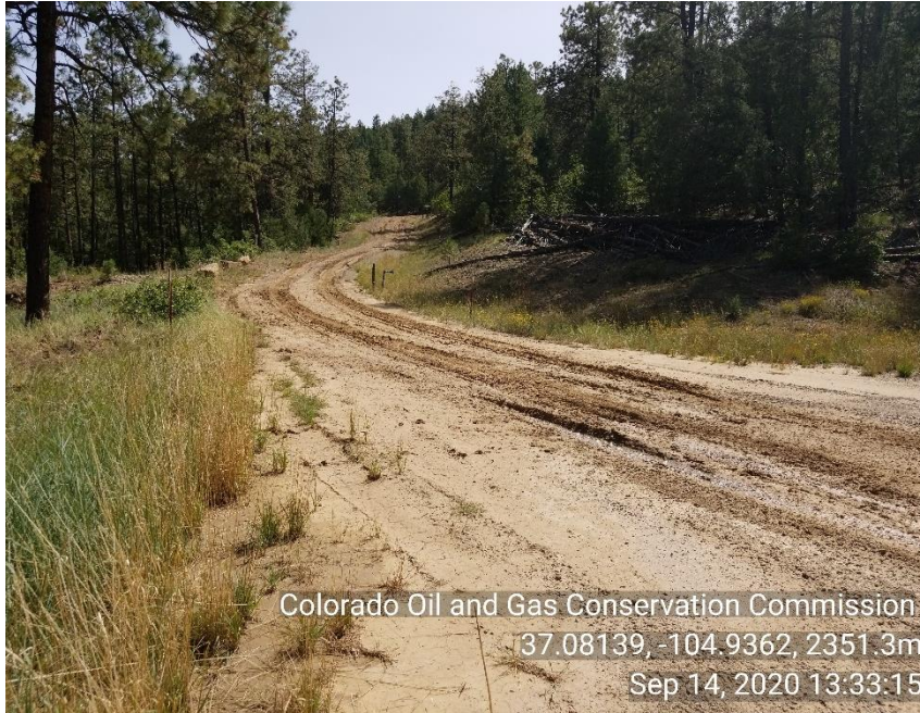
Photo 13 access road stormwater issues sediment being carried down road off location.
