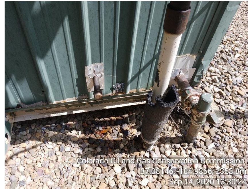
Photo 8 Stained soil from active leak in separator.
