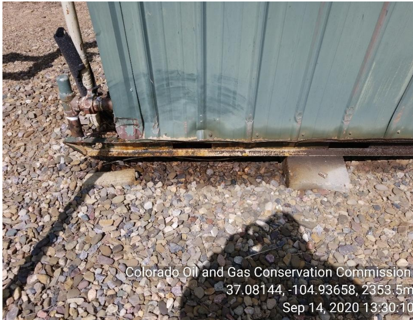
Photo 7 stained soil from active leak in separator
