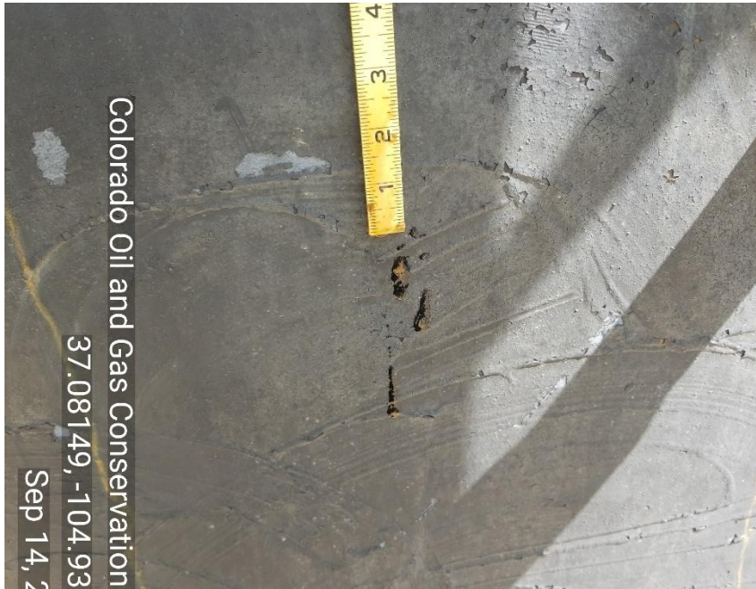
Photo 15 Approx.. 3in of what appears to be non E&P waste in 30bbl produced water tank.
