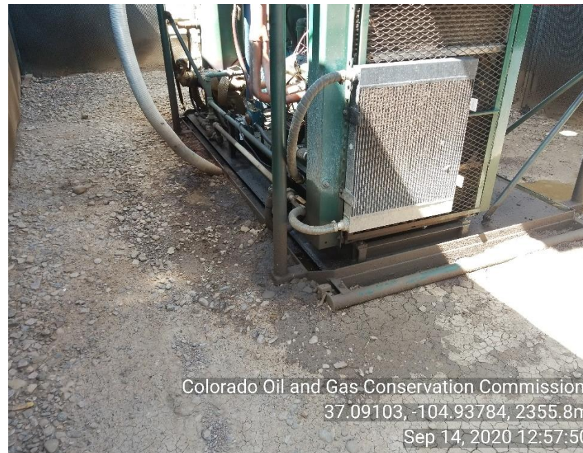
Photo 2 Stained soil around Liquid ring
