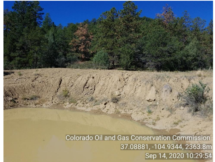
Photo 6 Stormwater running into production pit due to failed location BMP's.
