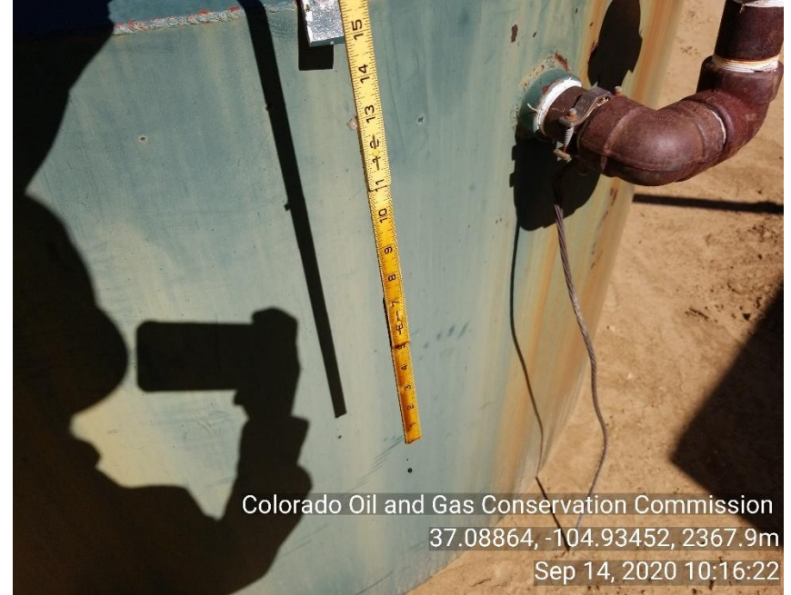
Photo 4 Approx 11 in of what appears to be non E&P waste in 30bbl produced water tank.
