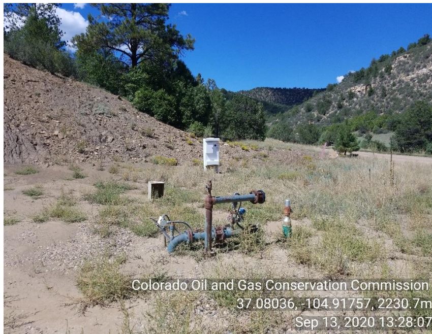
Photo 3 Well is TA. Risers not LOTO. Unused equipment risers and electric equipment. Weeds on location.
