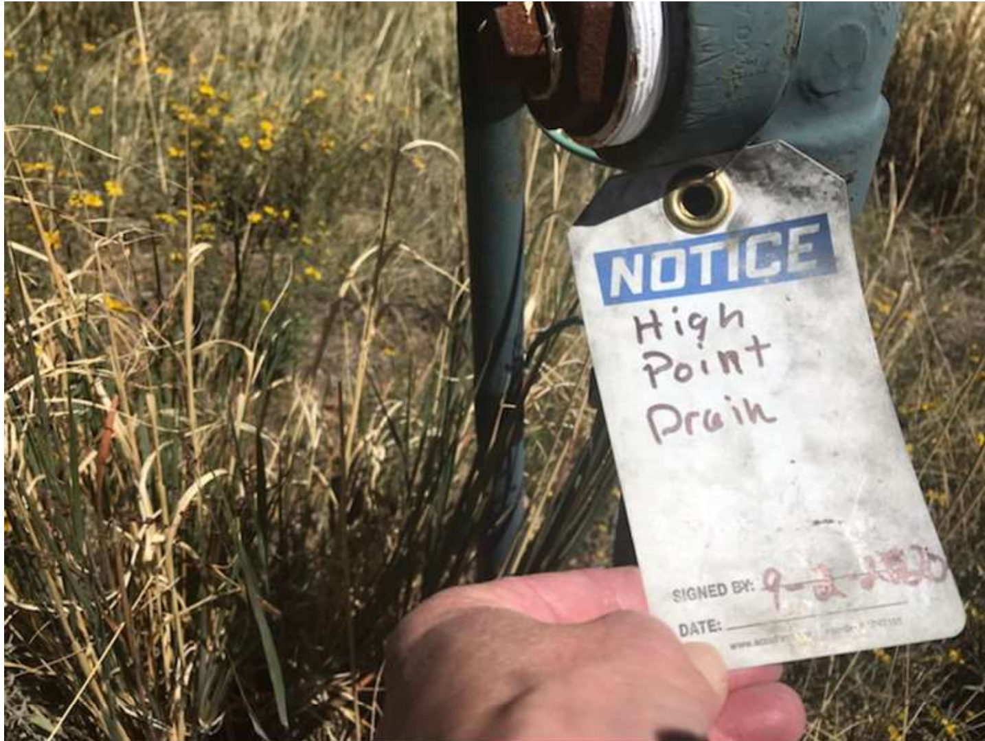
PHOTO 4: (1) RISER IS A LOW POINT DRAIN AND IS IN USE. (1) RISER IS A HIGH POINT DRAIN IN USE. THE RISER'S WERE LABLED WITH A TAG AND WITH A MARKER PIN AS TO THE FUNCTION FOR CLARITY.
