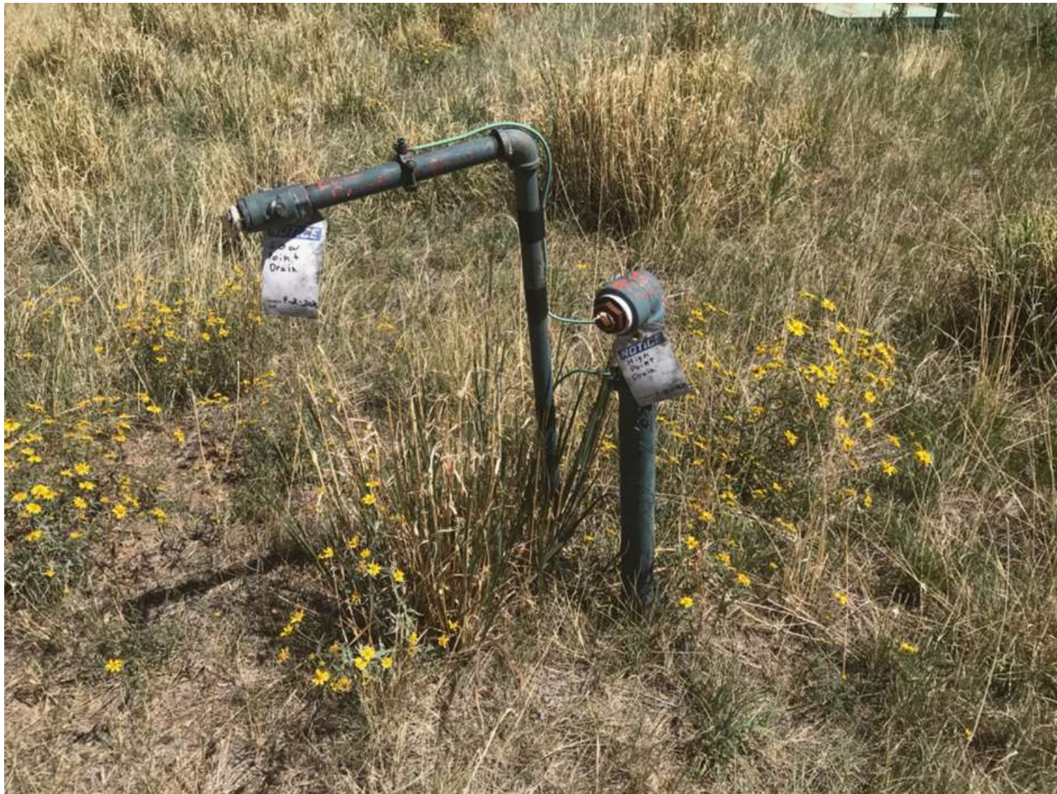
PHOTO 1: (1) RISER IS A LOW POINT DRAIN AND IS IN USE. (1) RISER IS A HIGH POINT DRAIN IN USE. THE RISER'S WERE LABLED WITH A TAG AND WITH A MARKER PIN AS TO THE FUNCTION FOR CLARITY.
