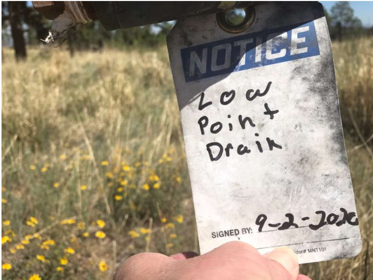
PHOTO 5: (1) RISER IS A LOW POINT DRAIN AND IS IN USE. (1) RISER IS A HIGH POINT DRAIN IN USE. THE RISER'S WERE LABELED WITH A TAG AND WITH A MARKER PIN AS TO THE FUNCTION FOR CLARITY.
