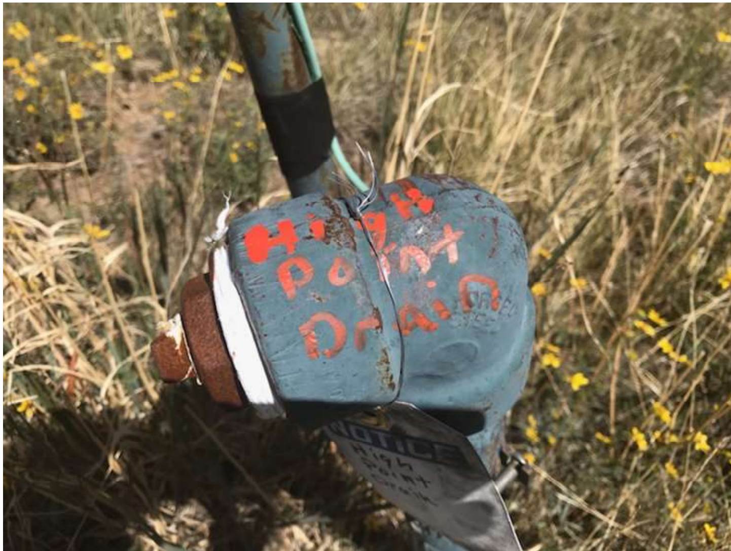
PHOTO 2: (1) RISER IS A LOW POINT DRAIN AND IS IN USE. (1) RISER IS A HIGH POINT DRAIN IN USE. THE RISER'S WERE LABLED WITH A TAG AND WITH A MARKER PIN AS TO THE FUNCTION FOR CLARITY.
