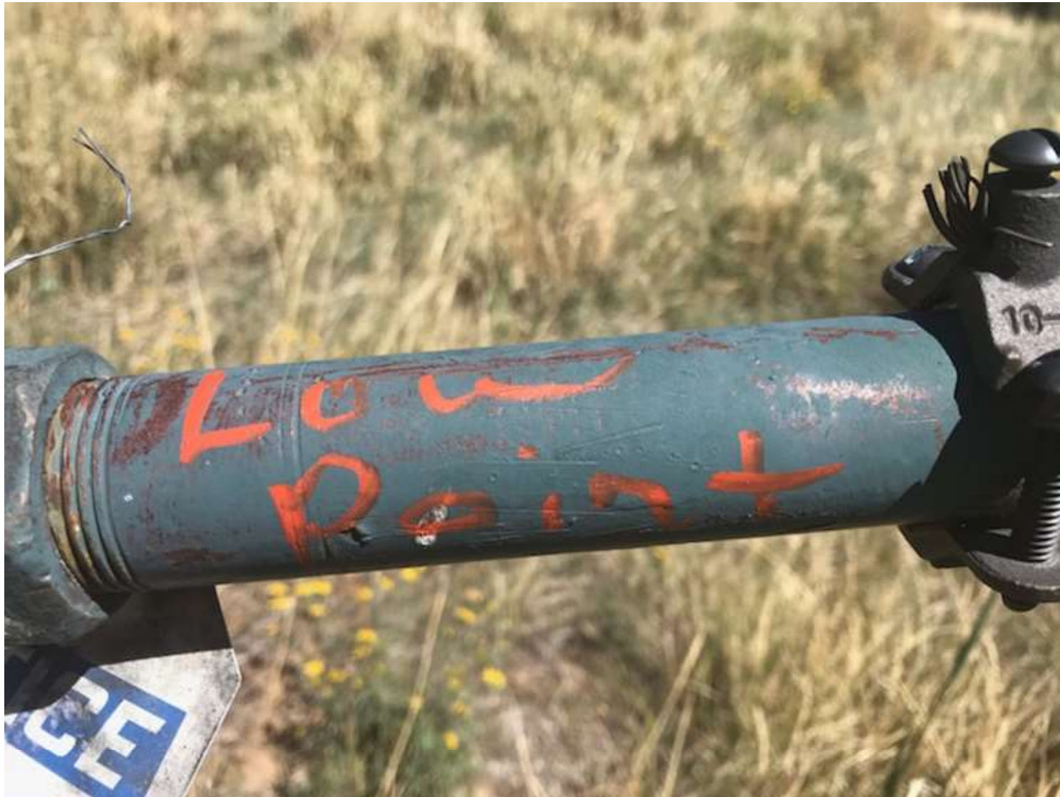
PHOTO 3: (1) RISER IS A LOW POINT DRAIN AND IS IN USE. (1) RISER IS A HIGH POINT DRAIN IN USE. THE RISER'S WERE LABLED WITH A TAG AND WITH A MARKER PIN AS TO THE FUNCTION FOR CLARITY.
