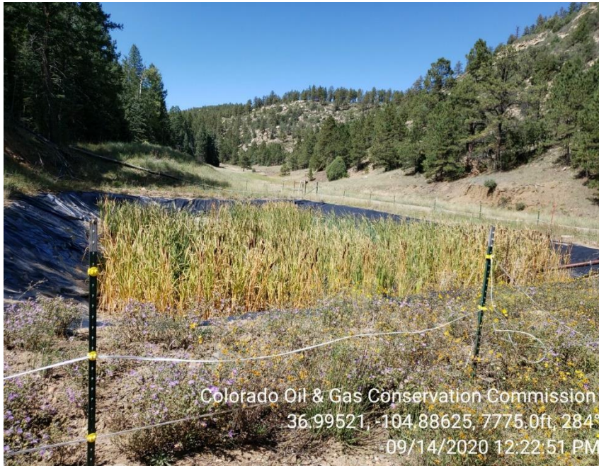
Photo 3 Pit has cat tails BMP 's Failing
