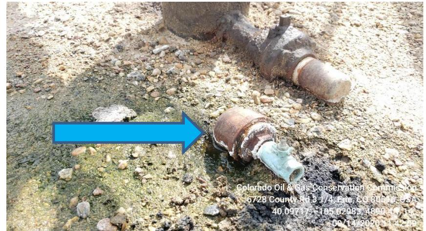
Photo 5 Braden head appears to have a leak from riser
