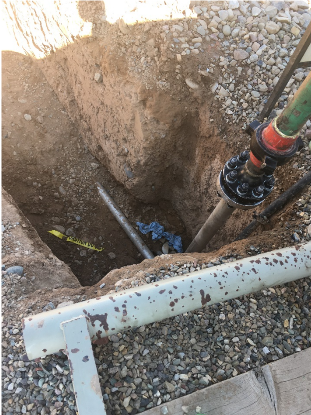
New 2" stainless steel dump line riser at separator
