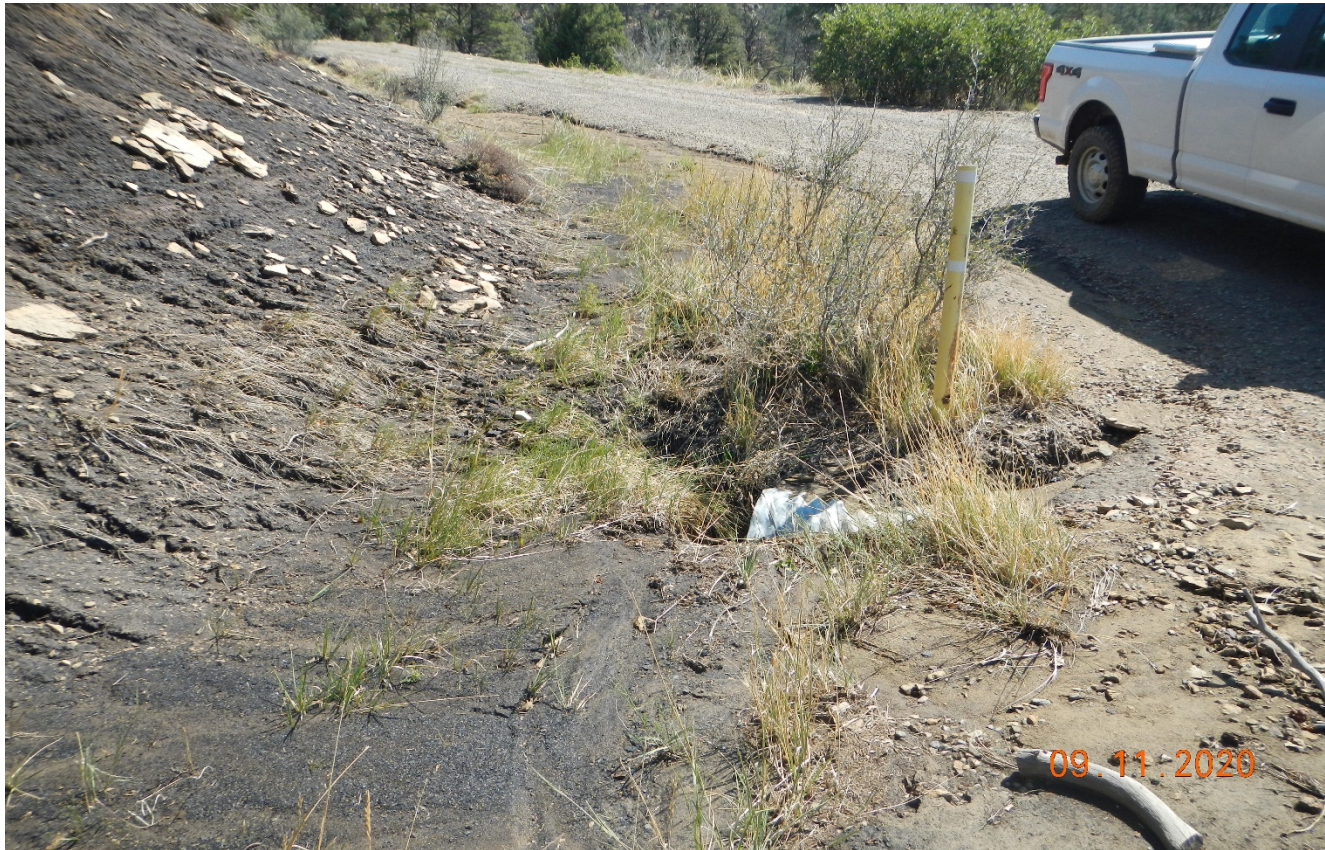
Photo 3. The culvert is filled in with sediment at beginning of the access road.
