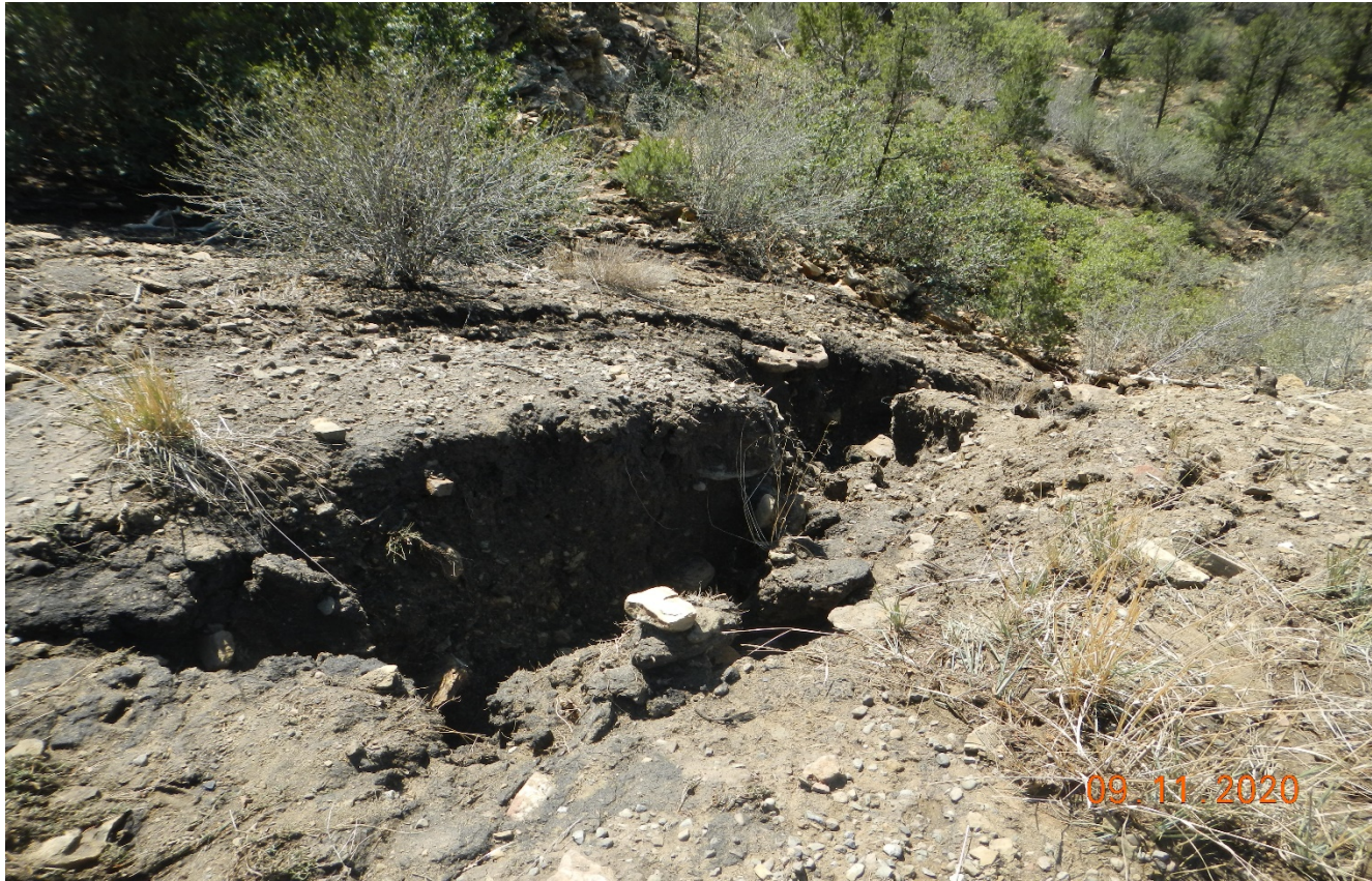
Photo 2. There is erosion occurring off the fill slope from stormwater flowing across the road shown in previous photo.
