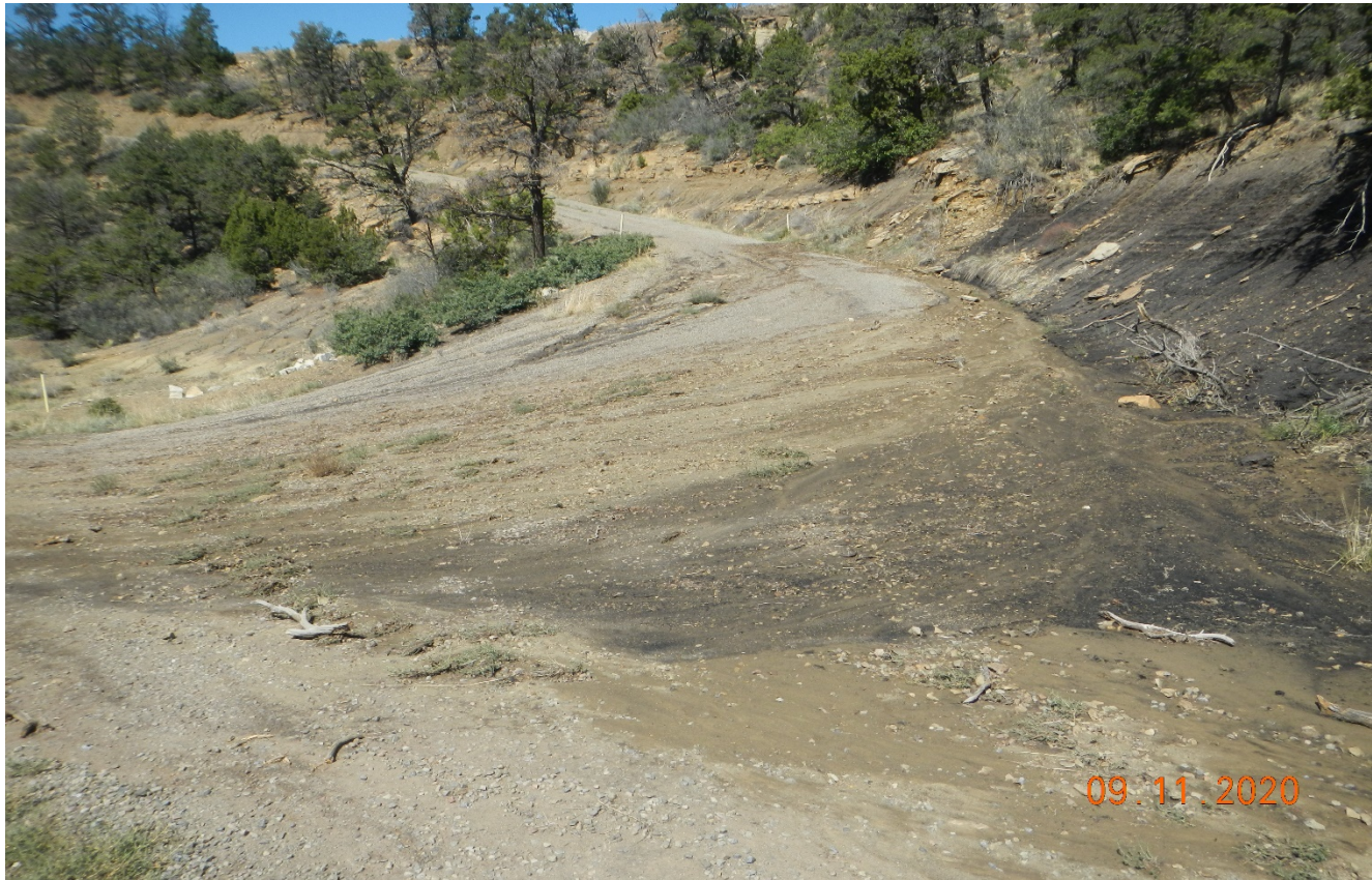
Photo 1. Facing northeast toward the access road. Stormwater is not flowing toward the culvert and is going across the road creating erosion shown in next photo.
