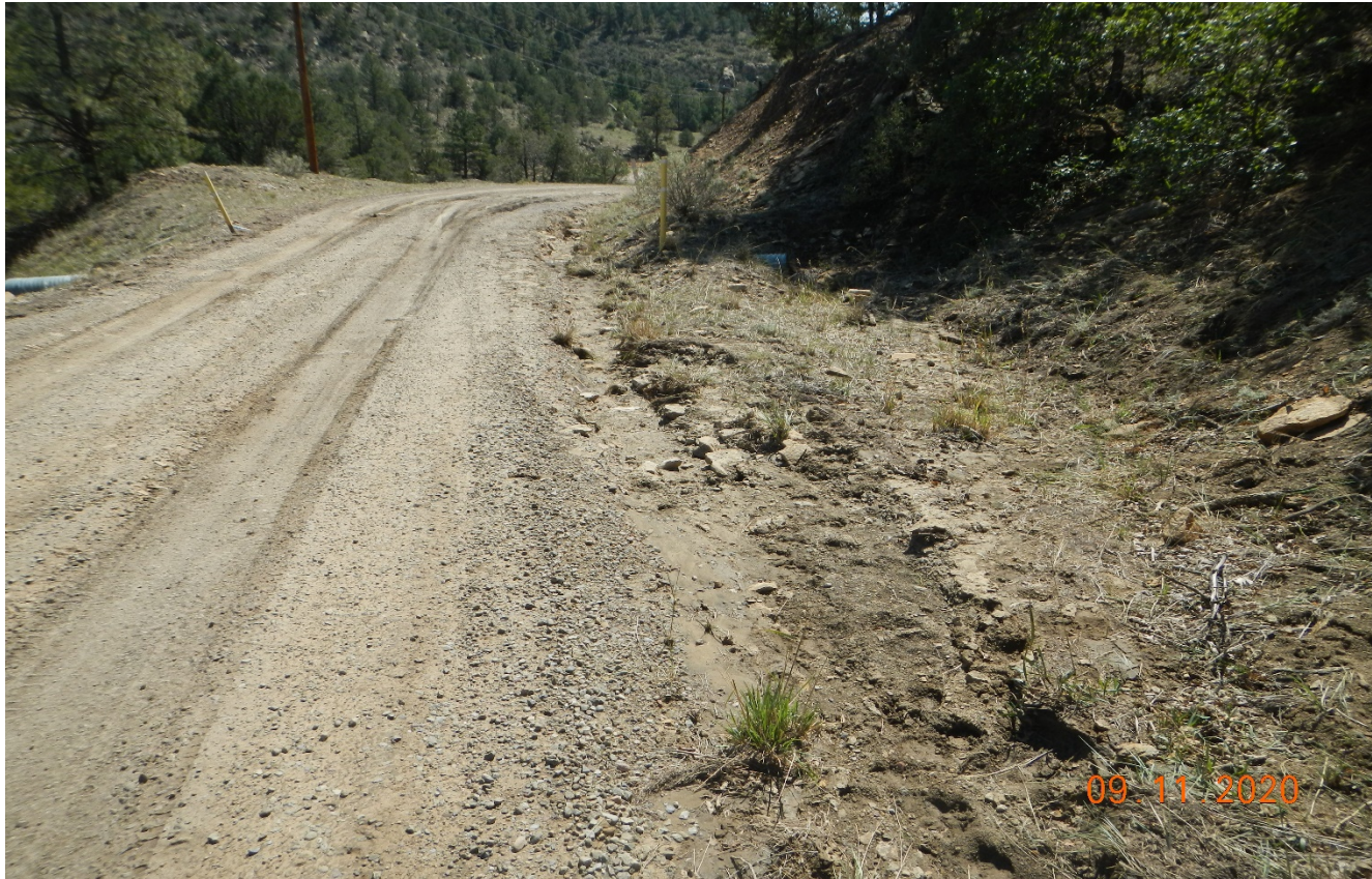
Photo 1. Facing southeast along the access road. Stormwater is not properly diverted toward the culvert in this area. Lat/Long:37.14697,-104.88575.
