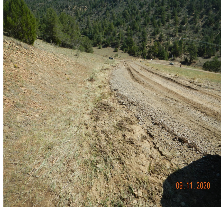
Photo 3. Facing back down the road where stormwater is flowing down the road causing the erosion shown in photo 1.
