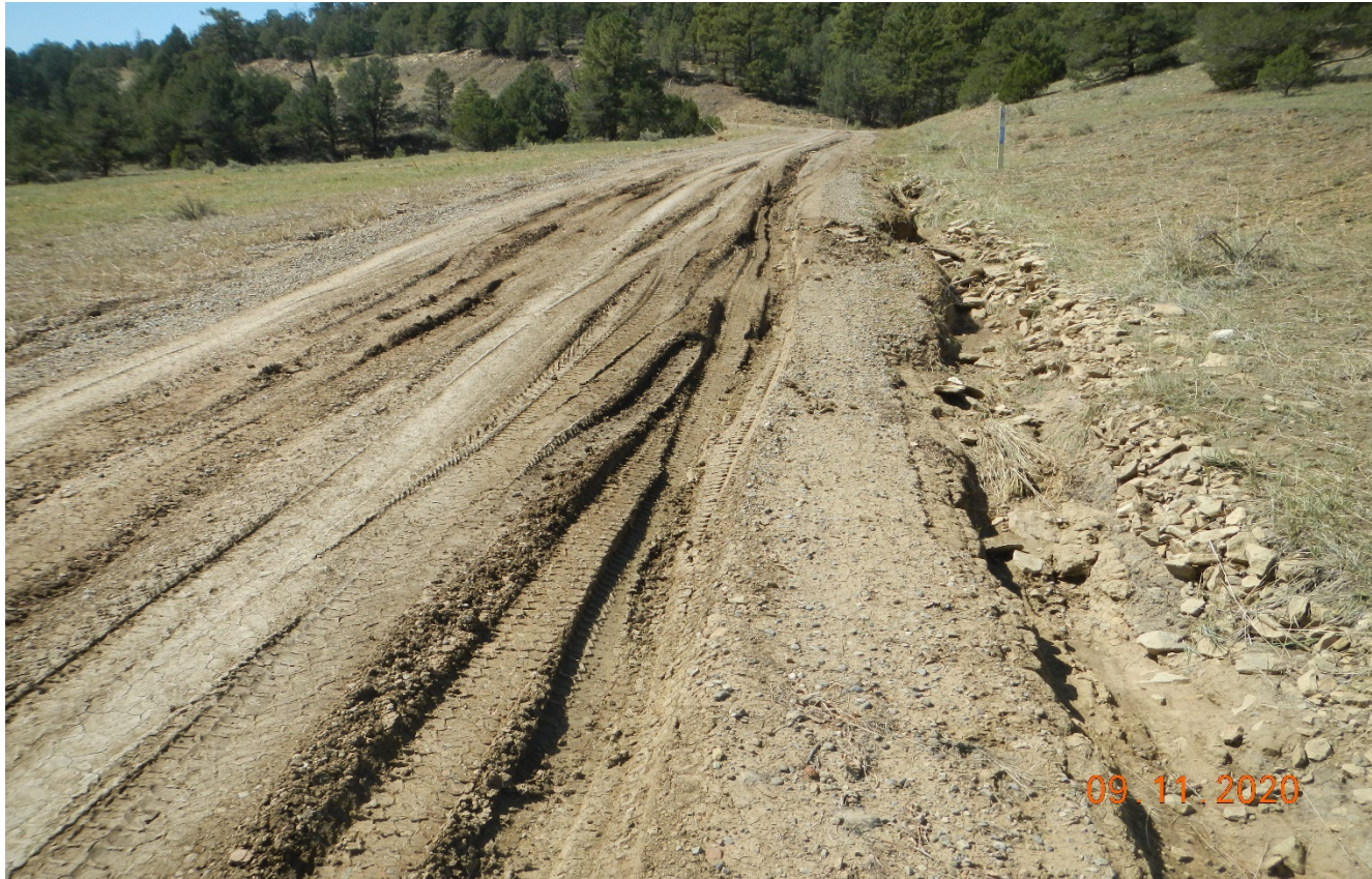
Photo 1. Facing southwest along the access road ascending the hillside. There is erosion occurring down the road and stormwater is not properly diverted toward the culvert up the road..
