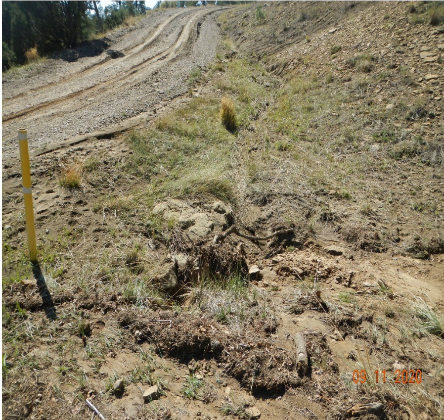
Photo 2. The culvert along the road has filled in with sediment causing stormwater to flow down the road.
