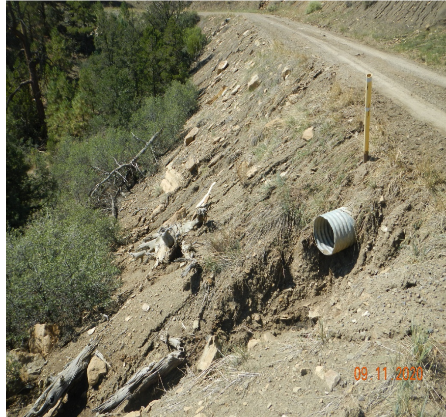
Photo 5. There is no culvert outlet protection which is causing erosion.
