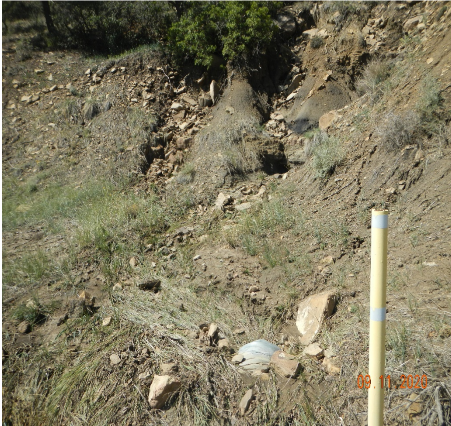
Photo 4. Another culvert further along the road is partially filled in with sediment.
