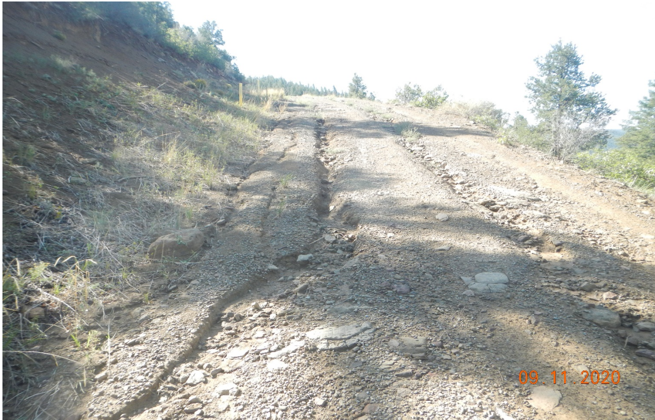
Photo 1. Facing south along the access road ascending the hillside. There is erosion occurring down the road and stormwater is not properly diverted toward the culvert.
