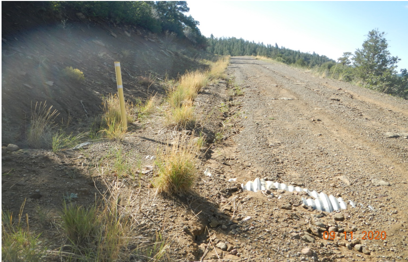
Photo 2. Stormwater is not properly diverted toward the culvert which is causing erosion of the road shown in previous photo.
