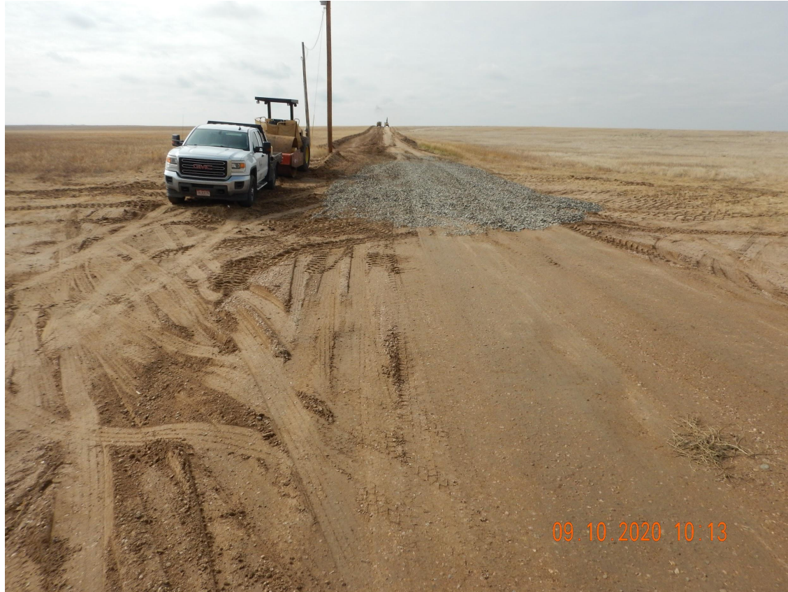
Photo 1. Photo taken from the entrance of the location off Hwy 14, facing South. Photo illustrates a tracking device BMP. At the time of this inspection, there were no track out issues observed.
