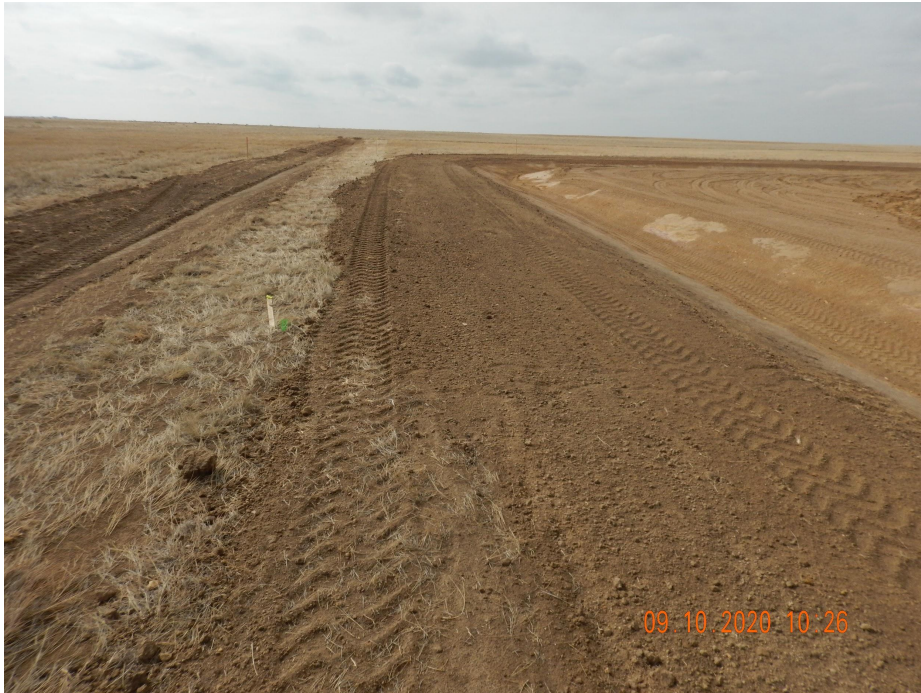
Photo 2. Photo taken from the eastern location, facing South. Photo illustrates two sets of ditch BMPs. The inner ditch BMP is directed to the northeastern retention area, while the outer ditch BMP appeared to be installed at the start of construction operations, controlling stormwater runoff and runon.
