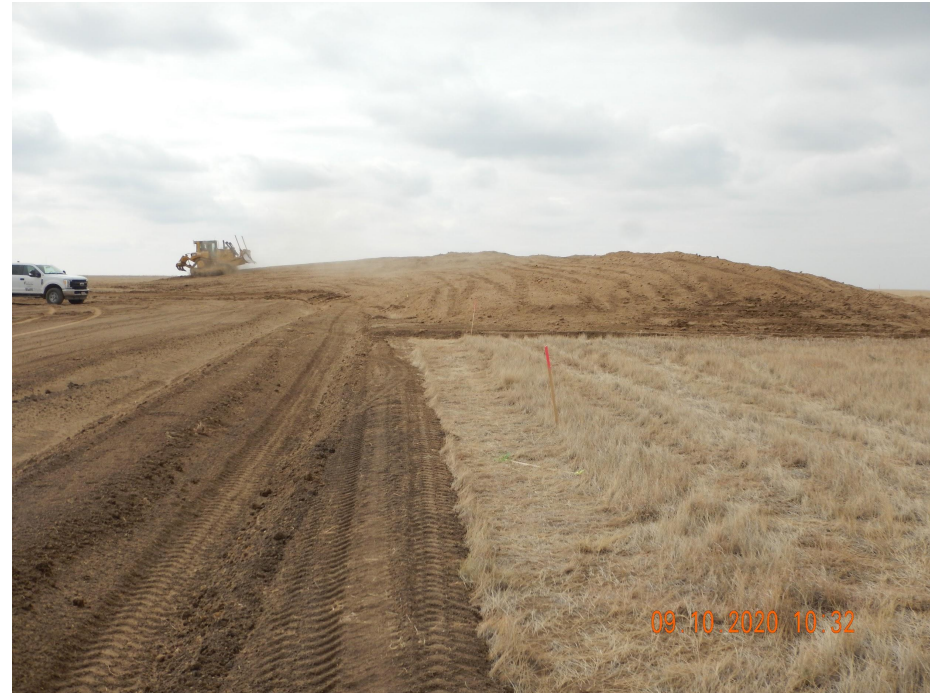
Photo 7. Photo taken from the western location, facing South. See comments under Photo 2. This photo also illustrates the topsoil stockpile along the southwestern location. At the time of this inspection, Operator was temporarily stabilizing the stockpile via equipment tracking.
