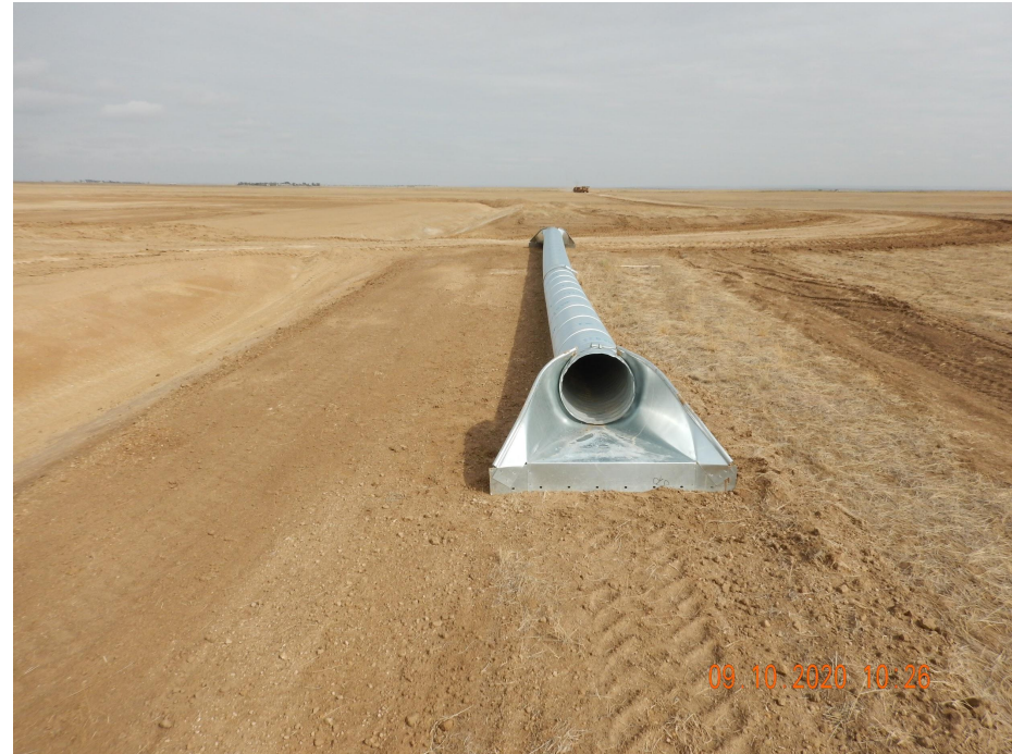
Photo 3. Photo taken from the eastern location, facing North. See comments under Photo 2. This photo also illustrates a culvert scheduled to be installed.
