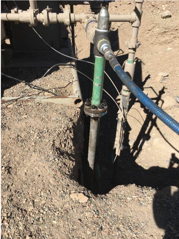
New 2" stainless steel dump line riser at separators
