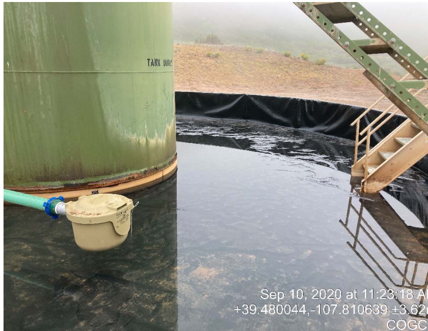
Follow up inspection shows new containment liner and no gravel
