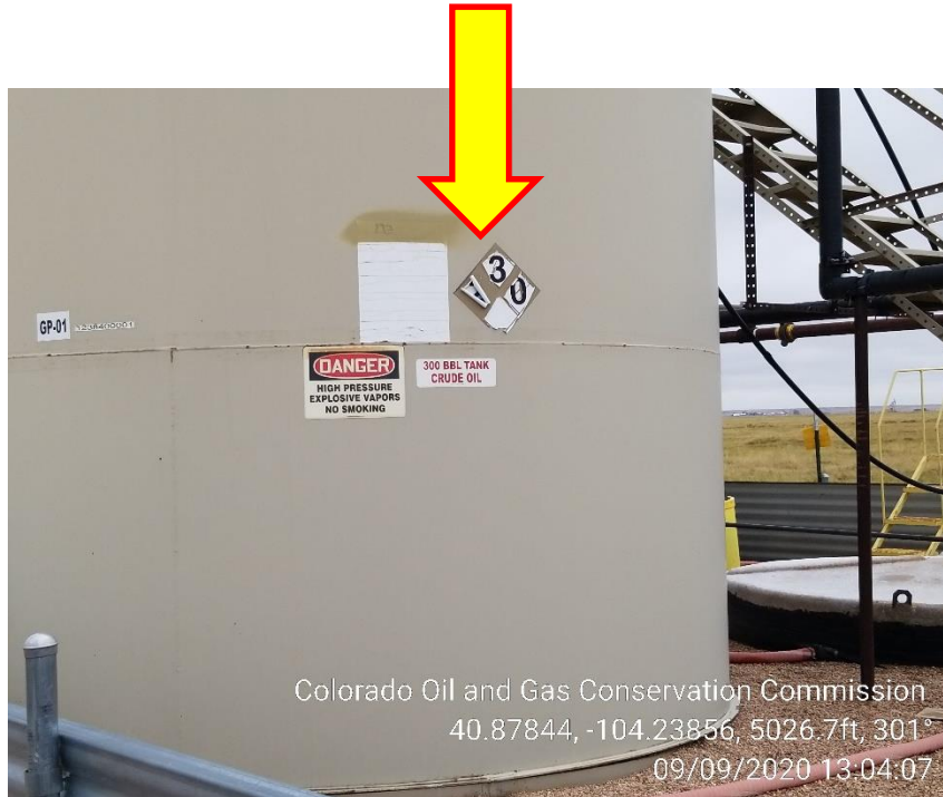
Photo 3 – 300 BBL Crude Oil Tank NFPA Label
