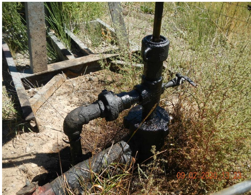
Well head and surrounding soil are stained and wet.
