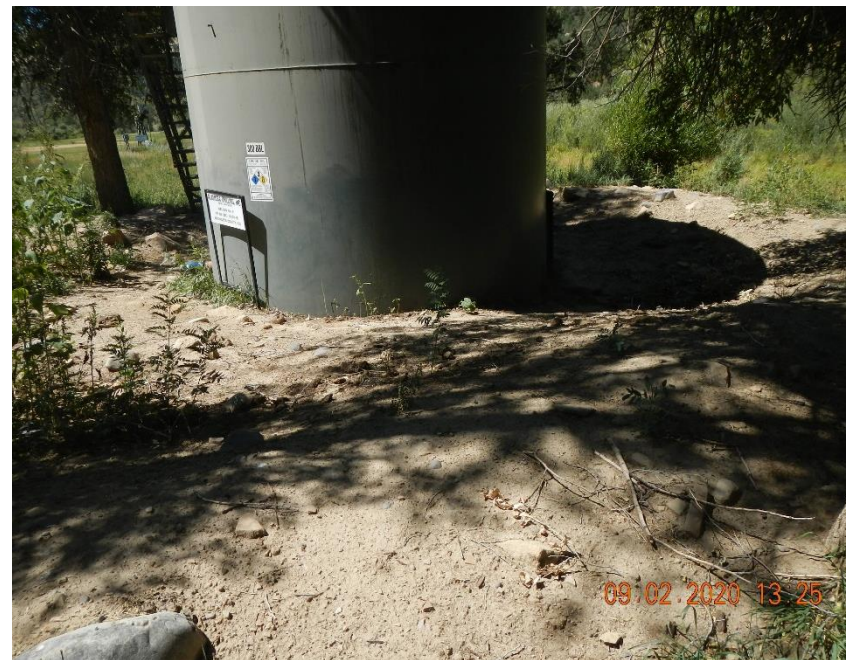
Ensure adequate capacity of secondary containment berm at Nielson #5 tank battery.
