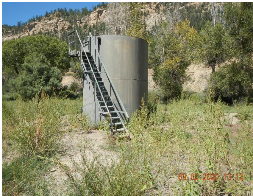
Weeds present within secondary containment berm.
