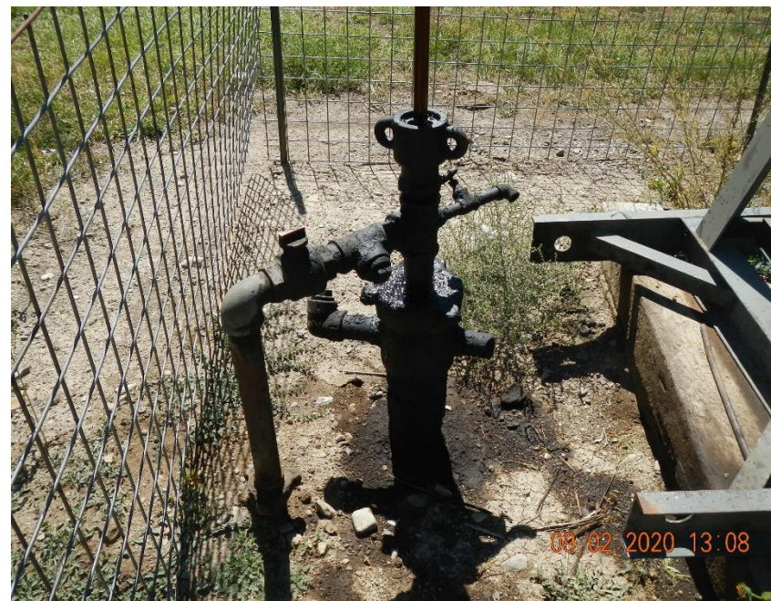
Staining around well head.
