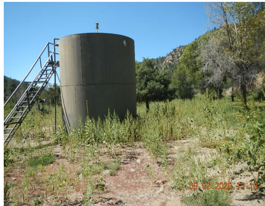
Nielson #4 crude oil AST. Weeds present within secondary containment berm.
