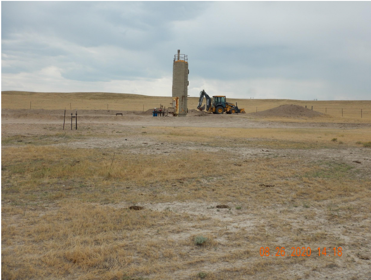
Photo 3. Photo taken from the tank battery location, facing Northwest. Photo illustrates the Operator is in process of decommissioning the tank battery with heavy equipment onsite.
