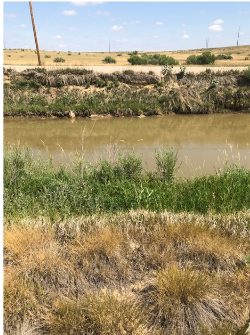
Photo 6: Larimer County Canal, north of location.
