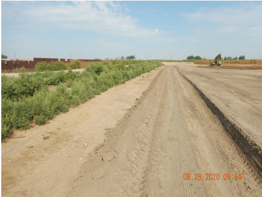
Photo 1. Photo taken from the southern location, facing West. Photo illustrates a ditch and berm BMP has been installed.
