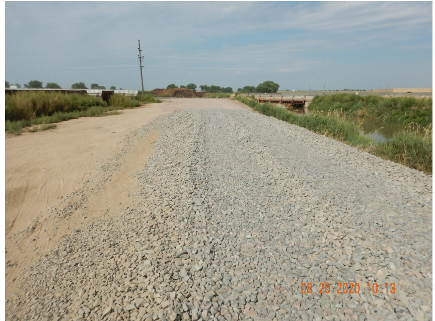
Photo 6. Photo taken from the entrance of the location off CR 39, facing West. Photo illustrates a vehicle tracking device BMP.
