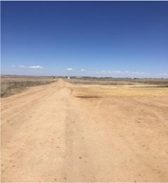
Photo 5 (below)-Access road, facing South
