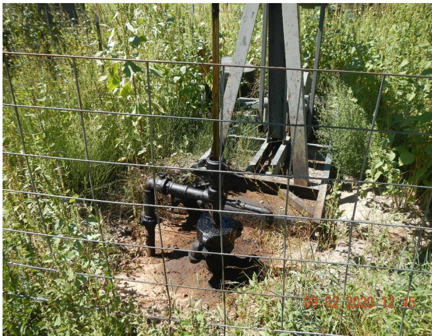
Well head is stained and wet.
