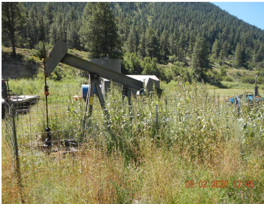
Weeds present near pump jack and within secondary containment for AST.
