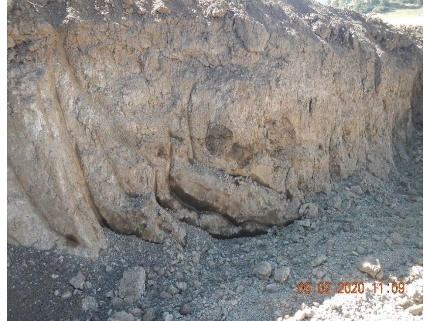
Impacted material in sidewall of excavation.
