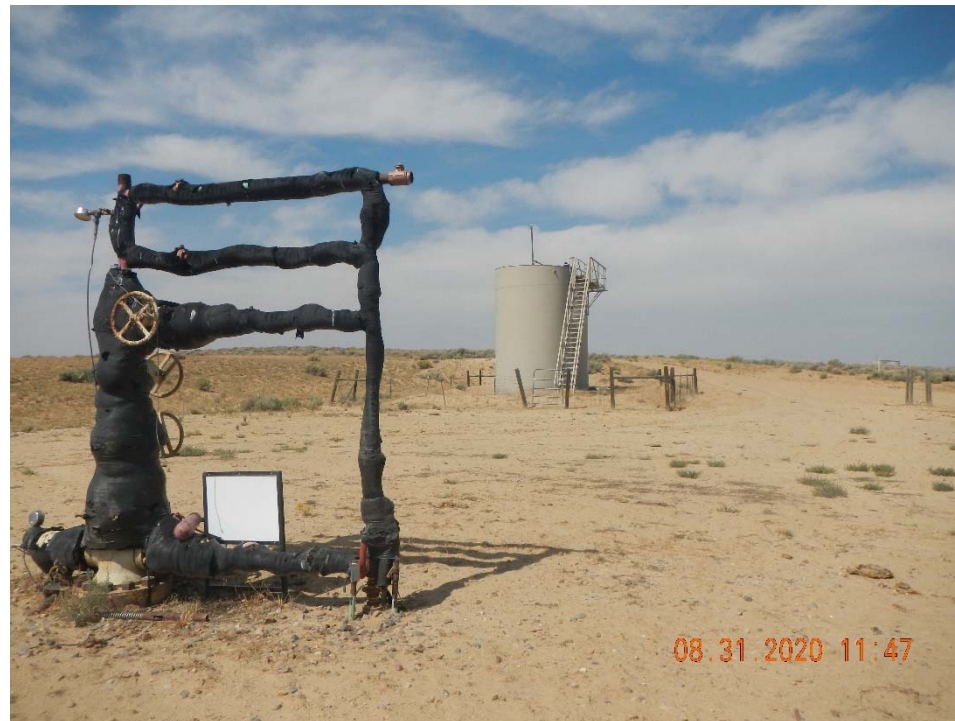
Photo 1. Overview of location taken facing north.
