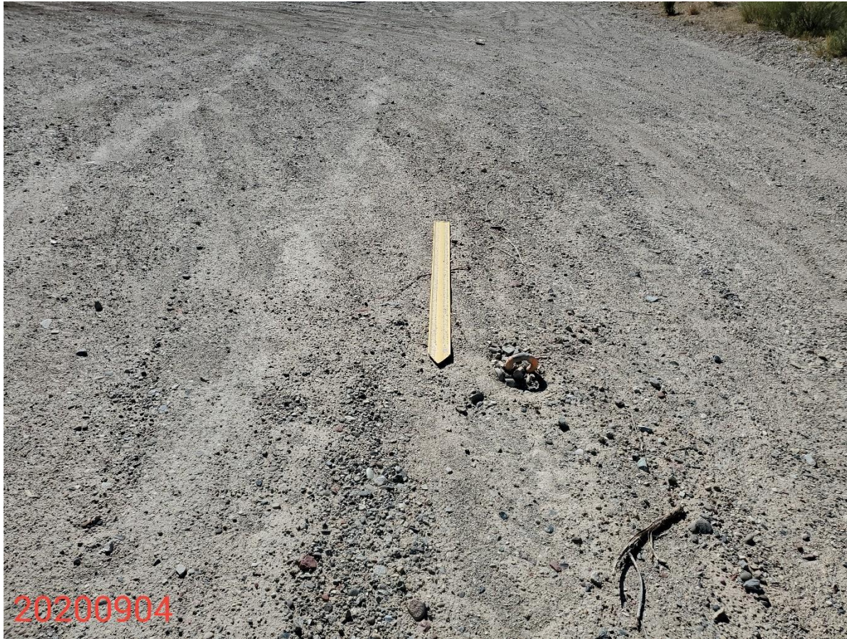
Photo 5: Photo shows the marker for southwestern guy line anchor is in disrepair.
