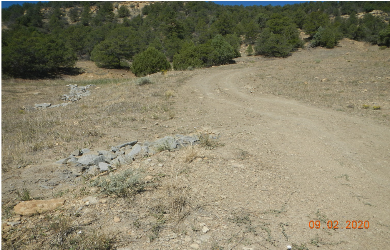
Photo 1. Facing northeast along the access road. Berms have been installed along the road with rock rip/rap.
