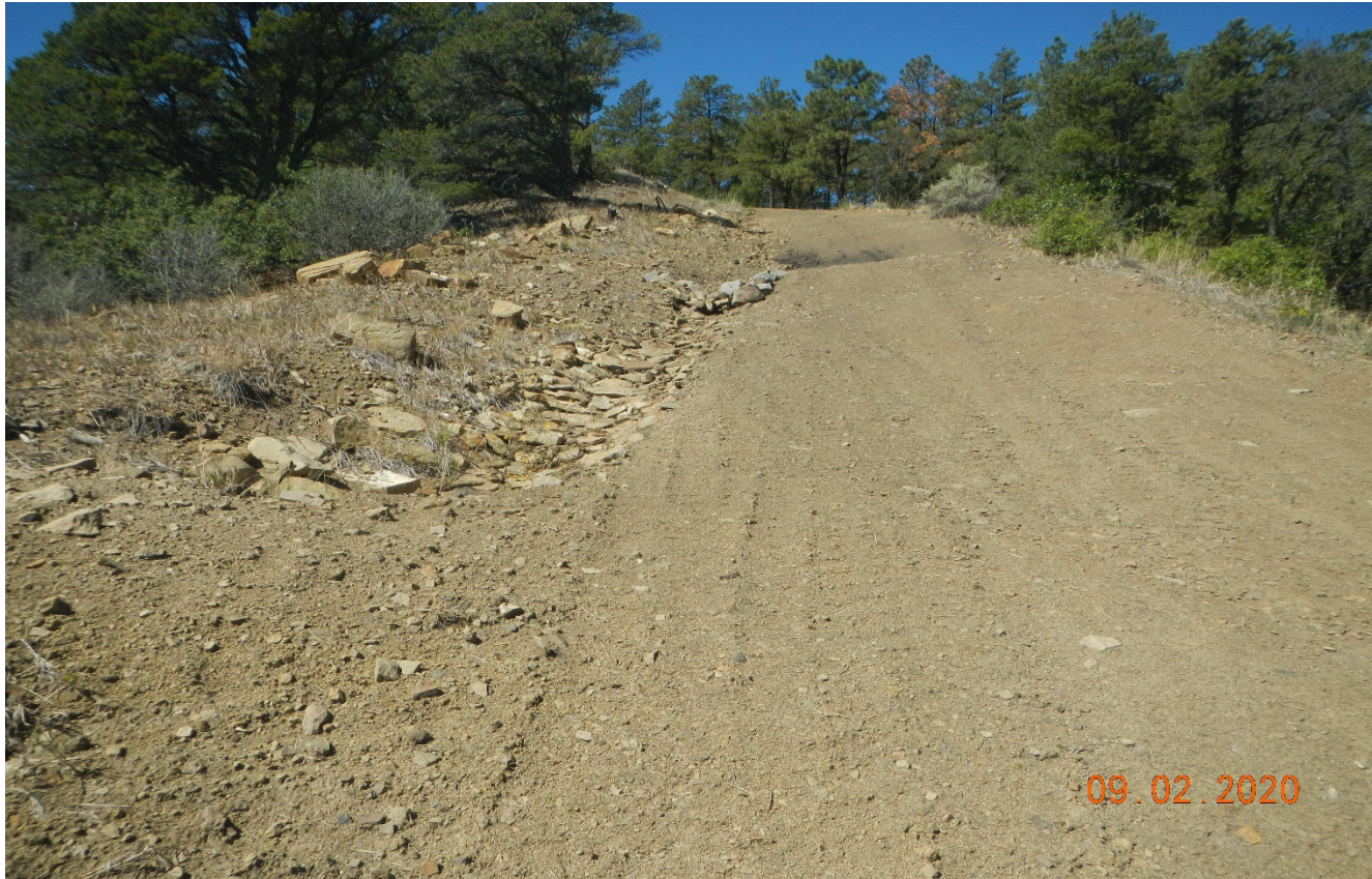
Photo 4. Facing west. Areas of erosion have been repaired and additional BMP's are installed.
