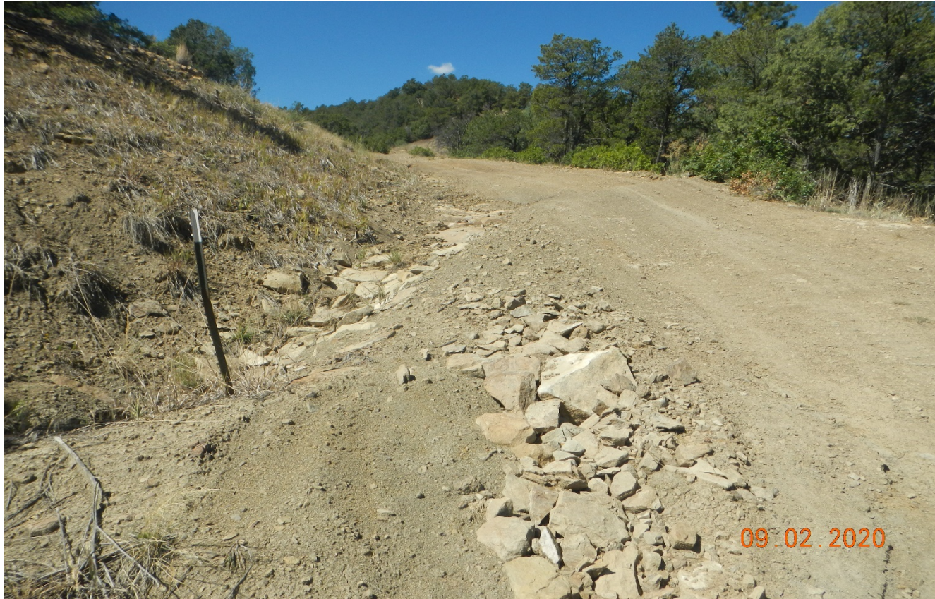
Photo 3. The erosion near the culvert has been repaired and a berm has been installed to direct stormwater towards the culvert.
