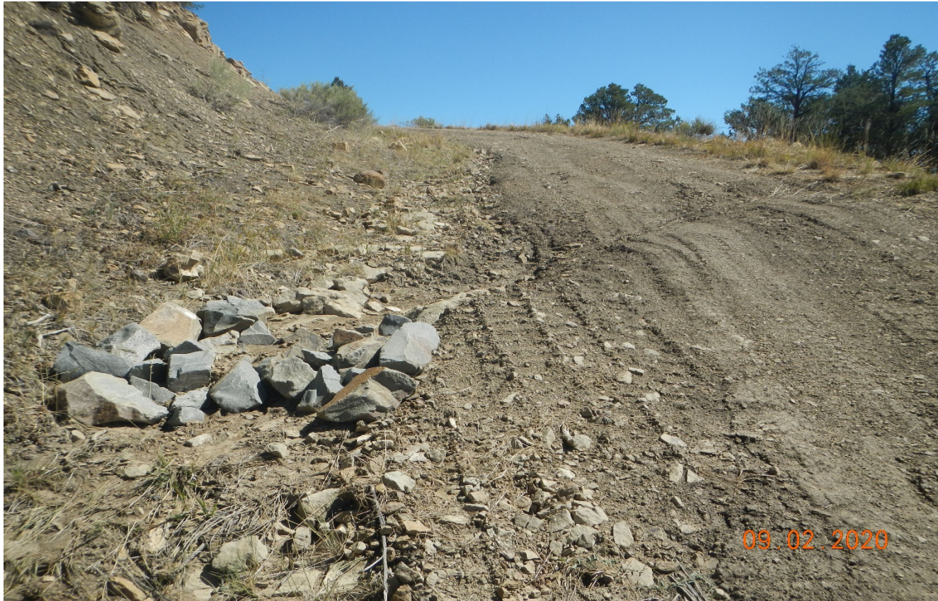
Photo 2. Facing northeast along the access road ascending the hill side. Additional berms have been installed along the road.
