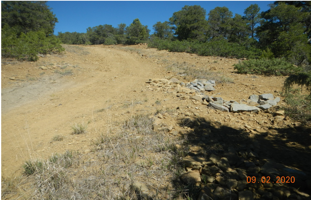
Photo 5. Facing north along the road. Areas of erosion have been repaired and additional BMP's are installed.
