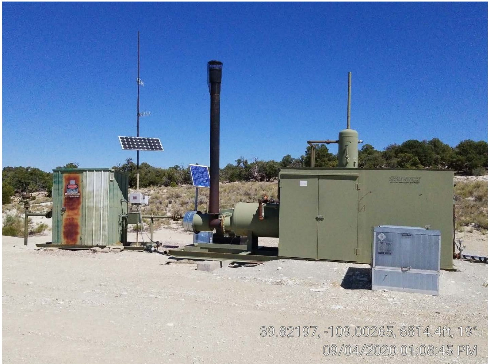
Photo 3. Meter building & separator.
