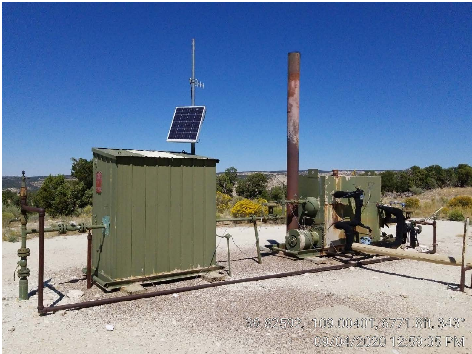
Photo 3. Meter building & separator.
