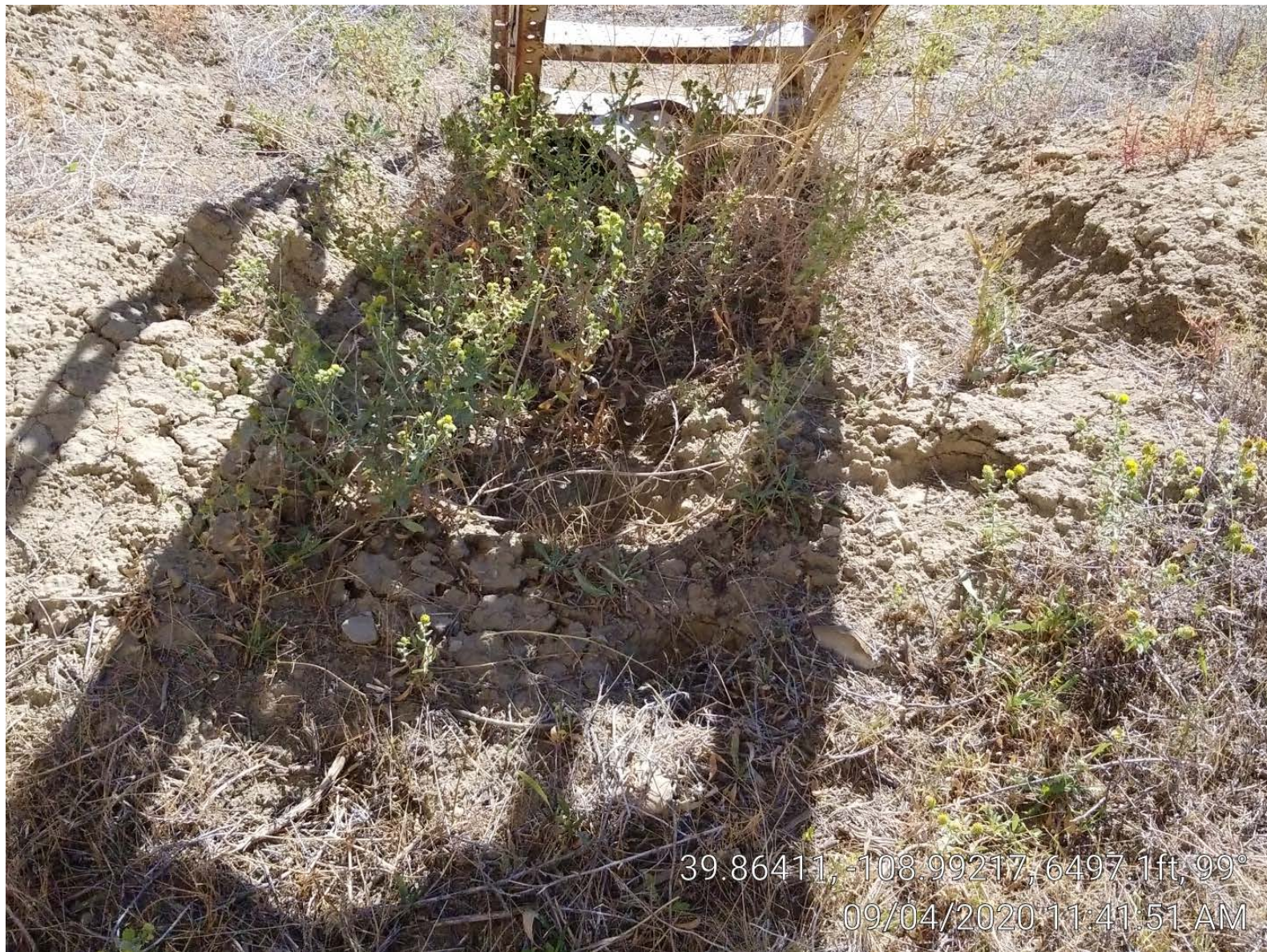
Photo 13. Tank berm missing under ladder.
