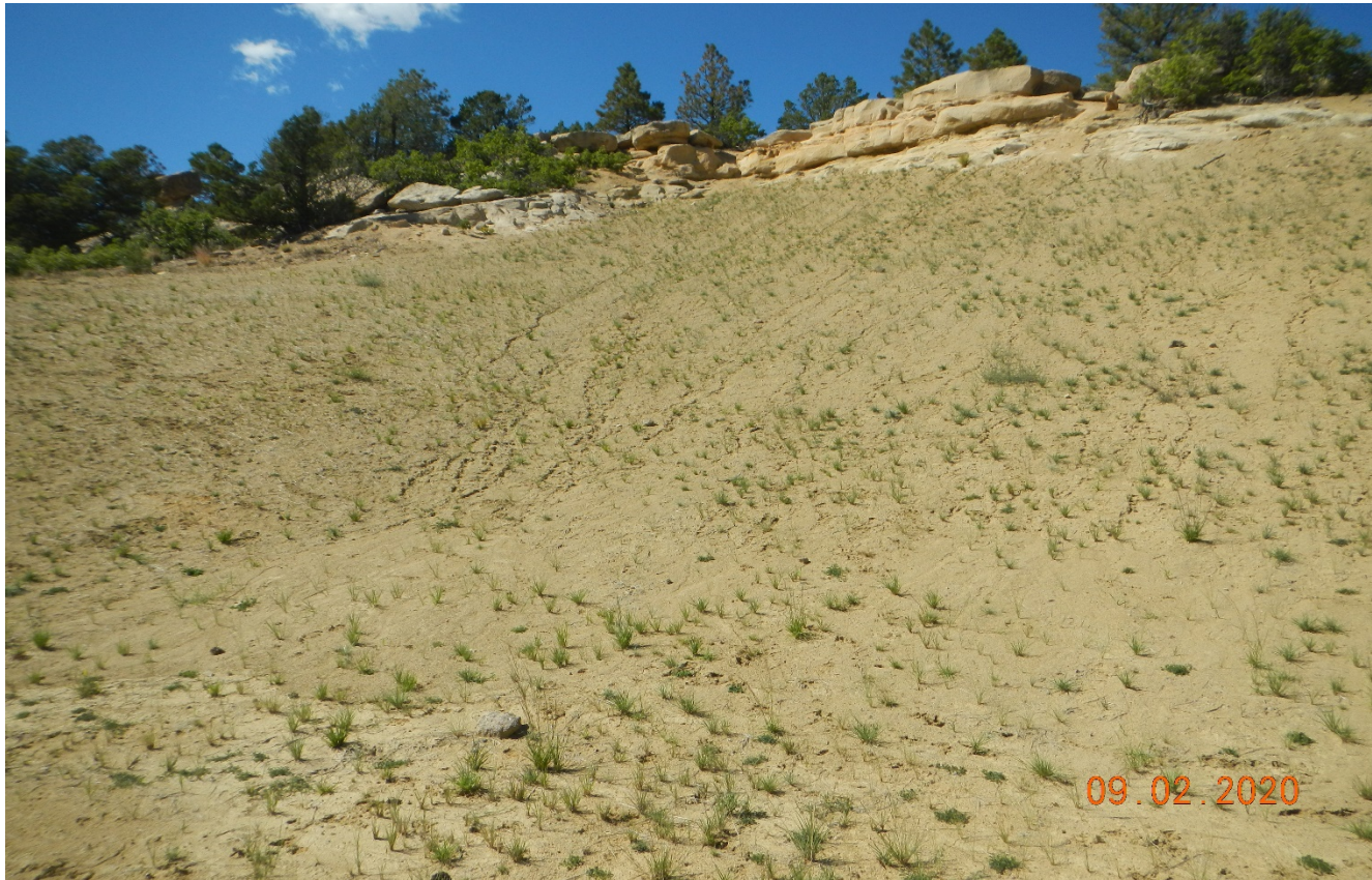
Photo 6. The cut slope is not stabilized and there is signs of erosion.
