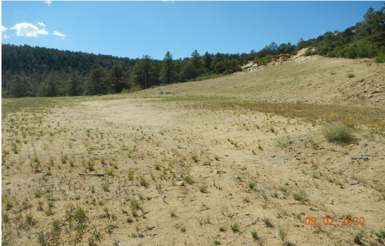
Photo 3. Facing west toward the location. The location has not been recontoured and reclaimed.
