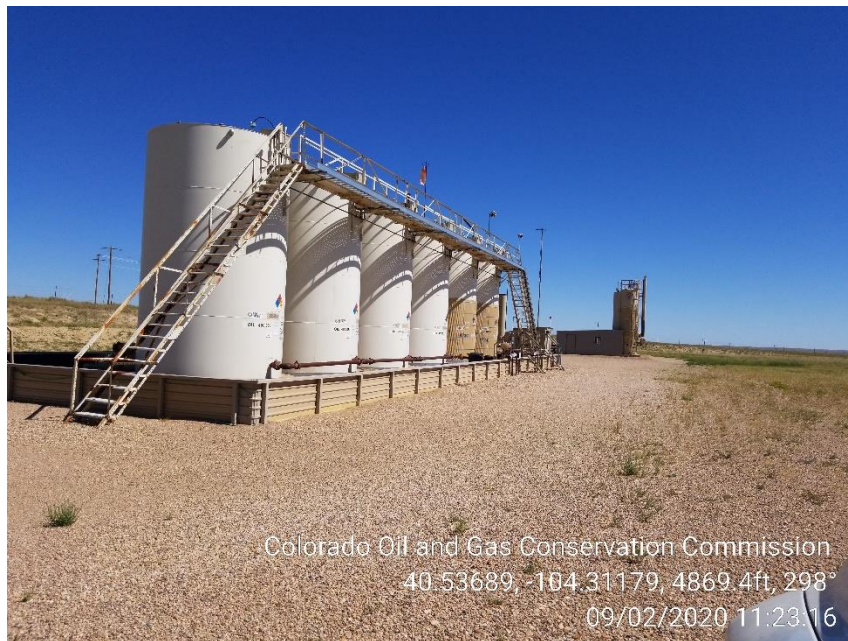
Photo 1 – Tank Battery
