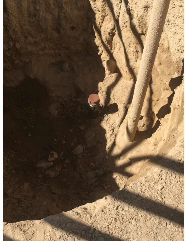
2" flowline abandoned in place. Threaded caps installed, Flowline cut 3' below grade
