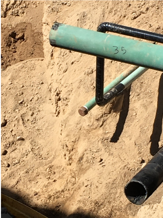
2" flowline abandoned in place. Threaded caps installed, Flowline cut 3' below grade
